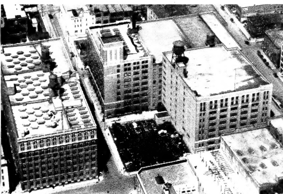
Offices and warehouses of FERRY'S SEEDS in Detroit cover twenty acres of floor space
