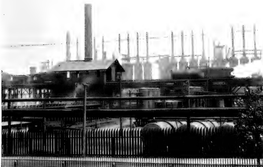
FIG. 1.—VIEW OF MODERN BY-PRODUCT COKE-OVEN PLANT WITH IRON FURNACE IN BACKGROUND.
