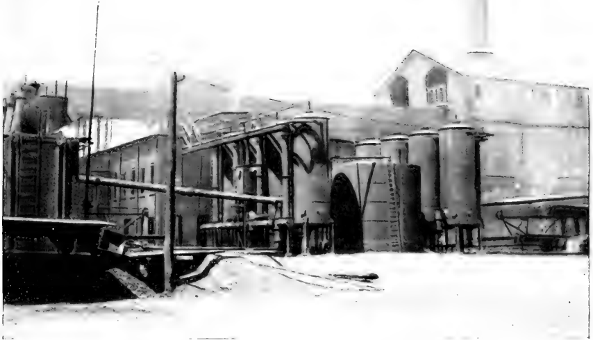
FIG. 1.—VIEW OF TAR AND LIQUOR CONDENSERS.
