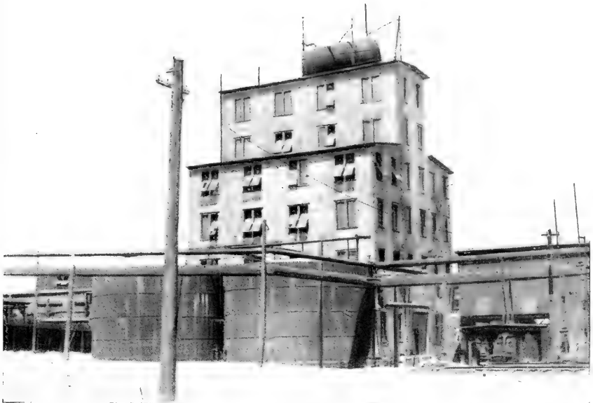
FIG. 2.—BY-PRODUCT HOUSE CONTAINING AMMONIA STILLS.
