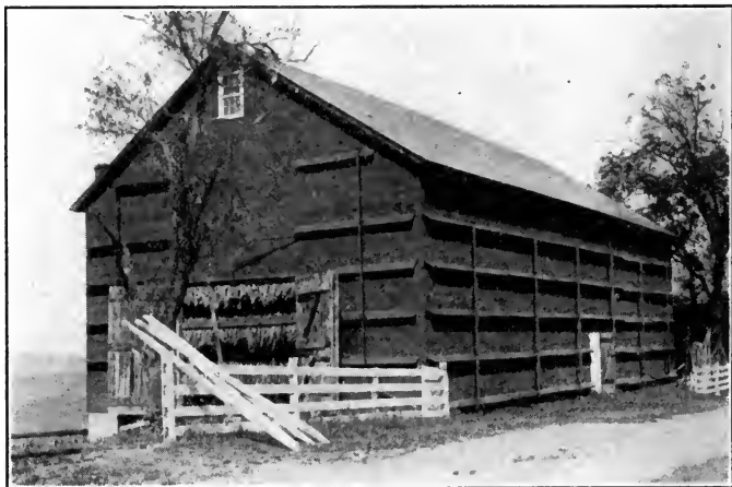
Fig. 149. A tobacco curing barn with horizontal ventilators. The method of hanging the leaves in the barn is shown.
