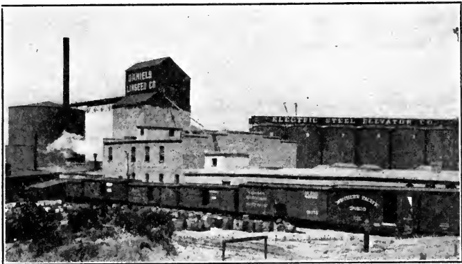
Fig. 83. A linseed oil mill, with steel tanks at the right for storing the flaxseed.
