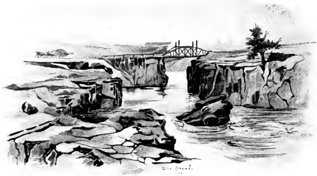
Eagle Rock Bridge. First one built across Snake River
