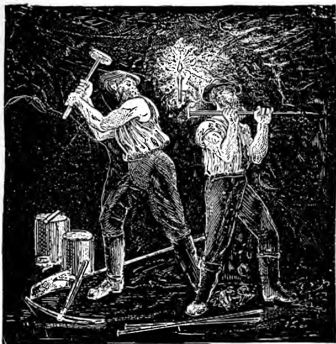
At the bottom of the shaft
