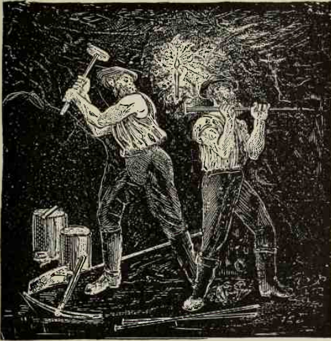
At the bottom of the shaft
