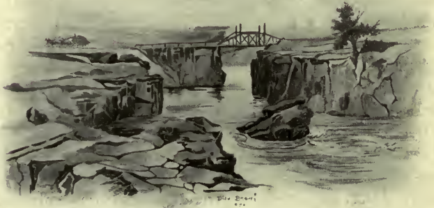
Eagle Rock Bridge. First one built across Snake River
