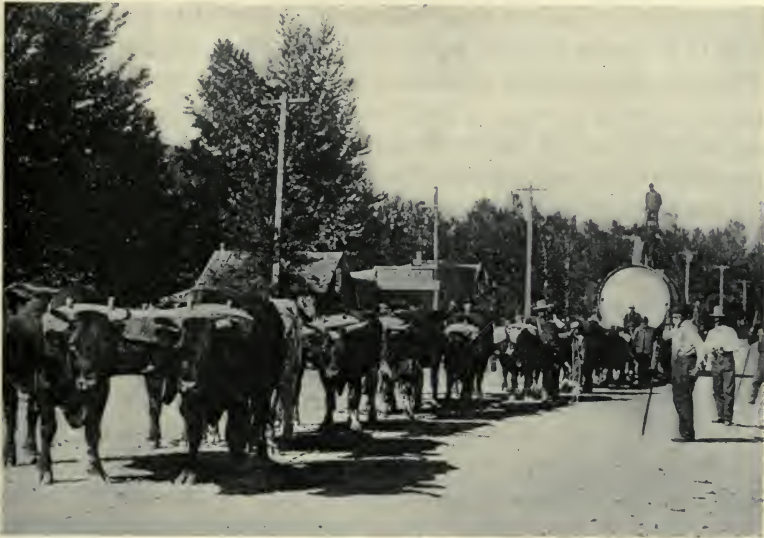
It took a herd of oxen to haul the gigantic boiler to the mines
