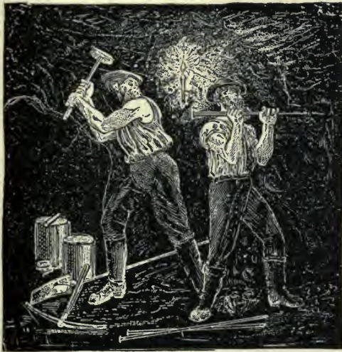
At the bottom of the shaft
