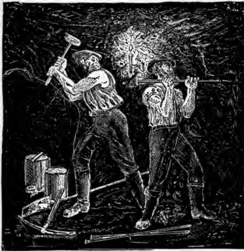
At the bottom of the shaft
