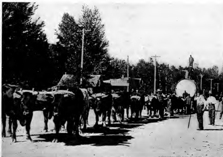
It took a herd of oxen to haul the gigantic boiler to the mines
