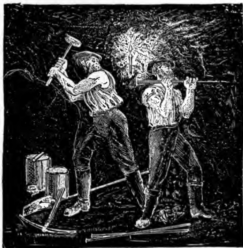
At the bottom of the shaft
