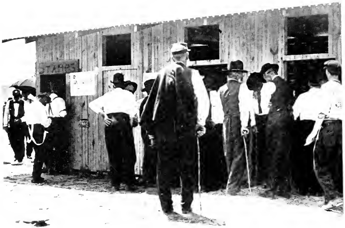
U. S. TEMPORARY POST OFFICE IN THE GREAT CAMP.
