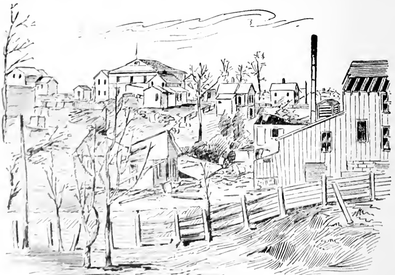
Rear of Mrs. Margaretha Burkhardt's Brewery, looking towards Turner Halle.
