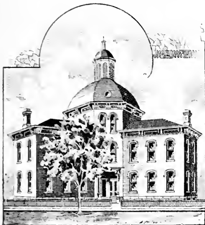
Perkins School House, corner West Exchange and Brewery Streets, Fifth Ward.
