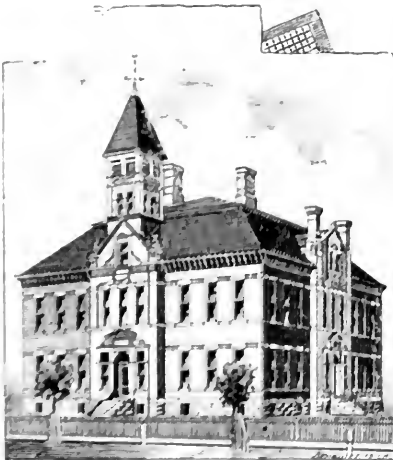
Henry School House, North Forge Street, Second Ward.
