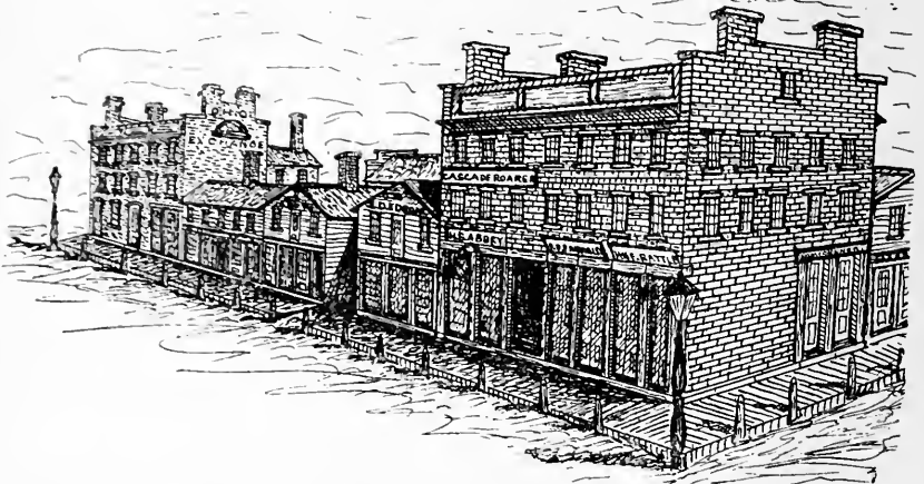
South side East Market Street, from Howard to Main, the "Old Stone Block," Ohio Exchange, etc., 1845. — Drawn from memory by the author.
