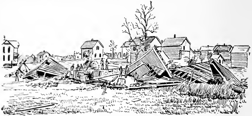
Residences of August C. Miller and Allen Coup, on Allyn Street, as left by the storm.
