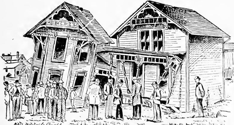
Residences of Alvin D. Alexander and Mrs. Kate O'Connell, 367 and 369 Carroll Street, after the storm.
