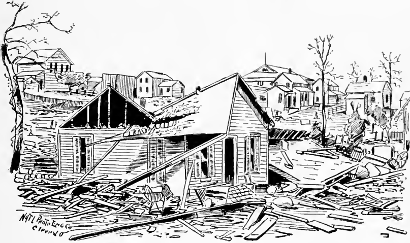
Wreck of Dormitory and other damage at Mrs. Margaretha Burkhardt's Brewery, Sherman Street.
