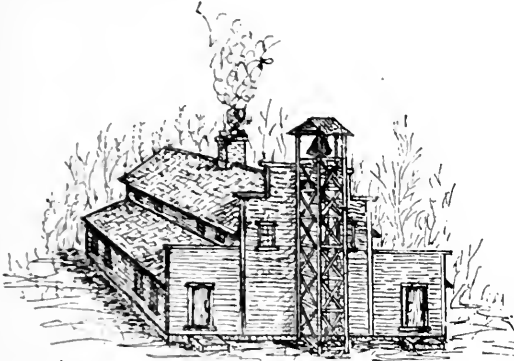
Akron's First High School Building—1847 to 1869, [On site of present Jennings School]
