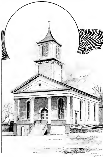
Original Baptist, late German Reformed Church, corner of South Broadway and Center Streets. Erected in 1836-37. Torn down in 1890.
