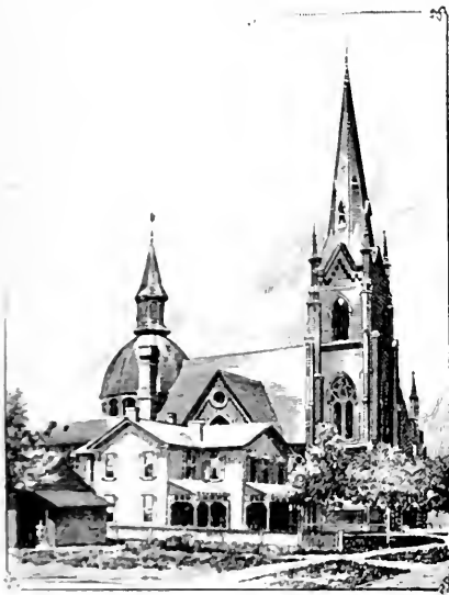
Trinity Lutheran Church and Parsonage—Prospect Street.
