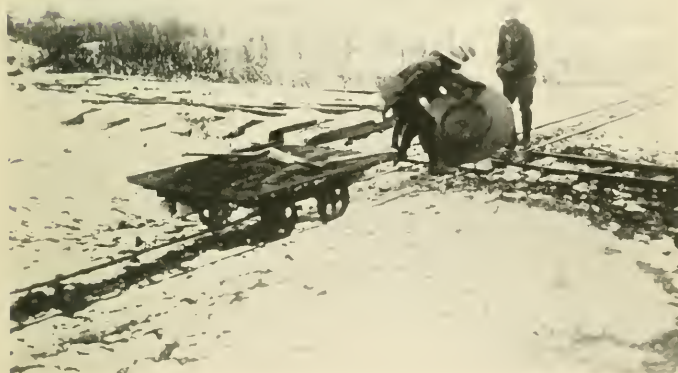
Placing a turntable on a narrow gauge railroad
