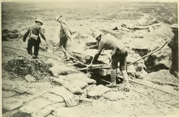
Narrow gauge construction
