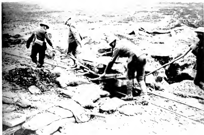
Narrow gauge construction
