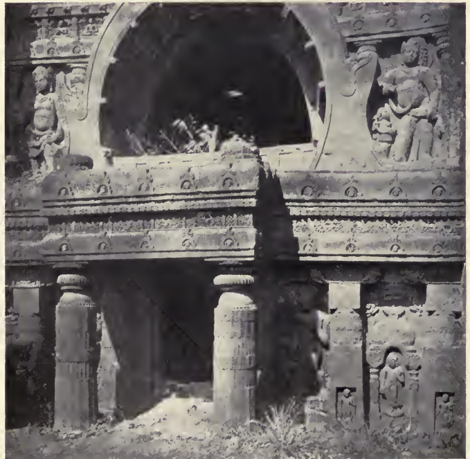
FACADE OF CHAITYA CAVE NO. 19 AT AJANTA.
