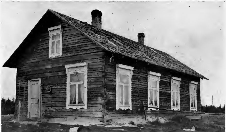
FIG. 8—A typical Finnish log cabin with windows which identify the nationality. The corners of the cabin are boxed off and the logs are squared, the squaring being done after the logs have been put in place. It represents a bit of Finnish mechanical skill. Toivola—"the place of hope"—Minn.
