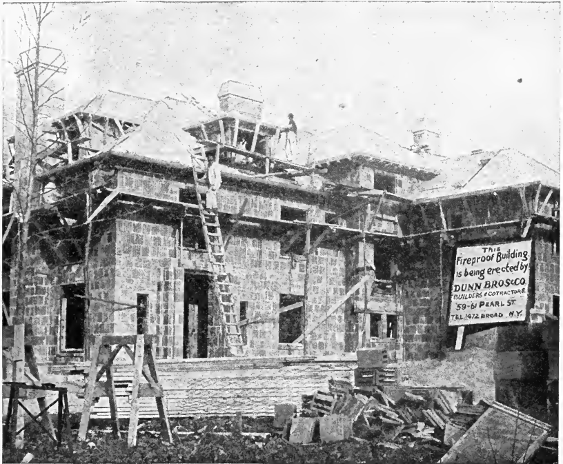
Fig. 71. A Tile Fireproof House, Roof, Walls, Floors and All of Hollow Tile
