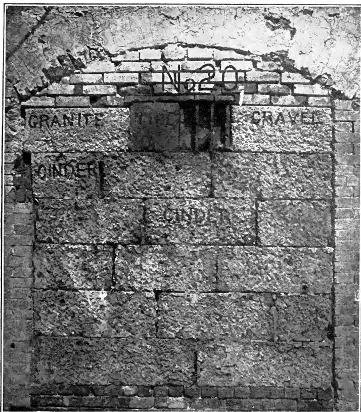
Fig. 117. Appearance After Test of Panel Containing Cinder-Concrete Beams
