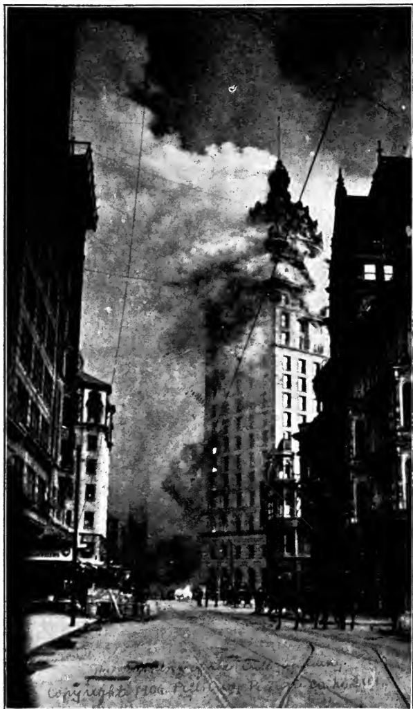
Fig. 26. Fire's Ingress via the Window Route
