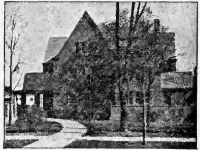
Fig. 65. Exterior Design for House, by Chicago Architects, That Would Fit Plans of House A
