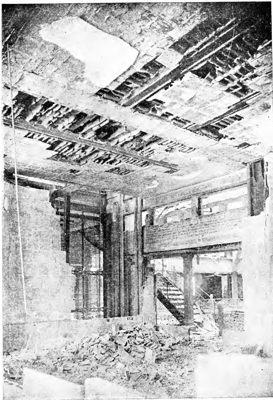
Fig. 26. The Effect of Fire Upon Too Thin and Dense Hollow Tile
