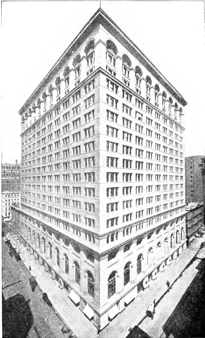
Fig. 31. The First National Bank, One of Chicago's Tall Office Buildings, as Well Fireproofed as any Specimen of its Kind
