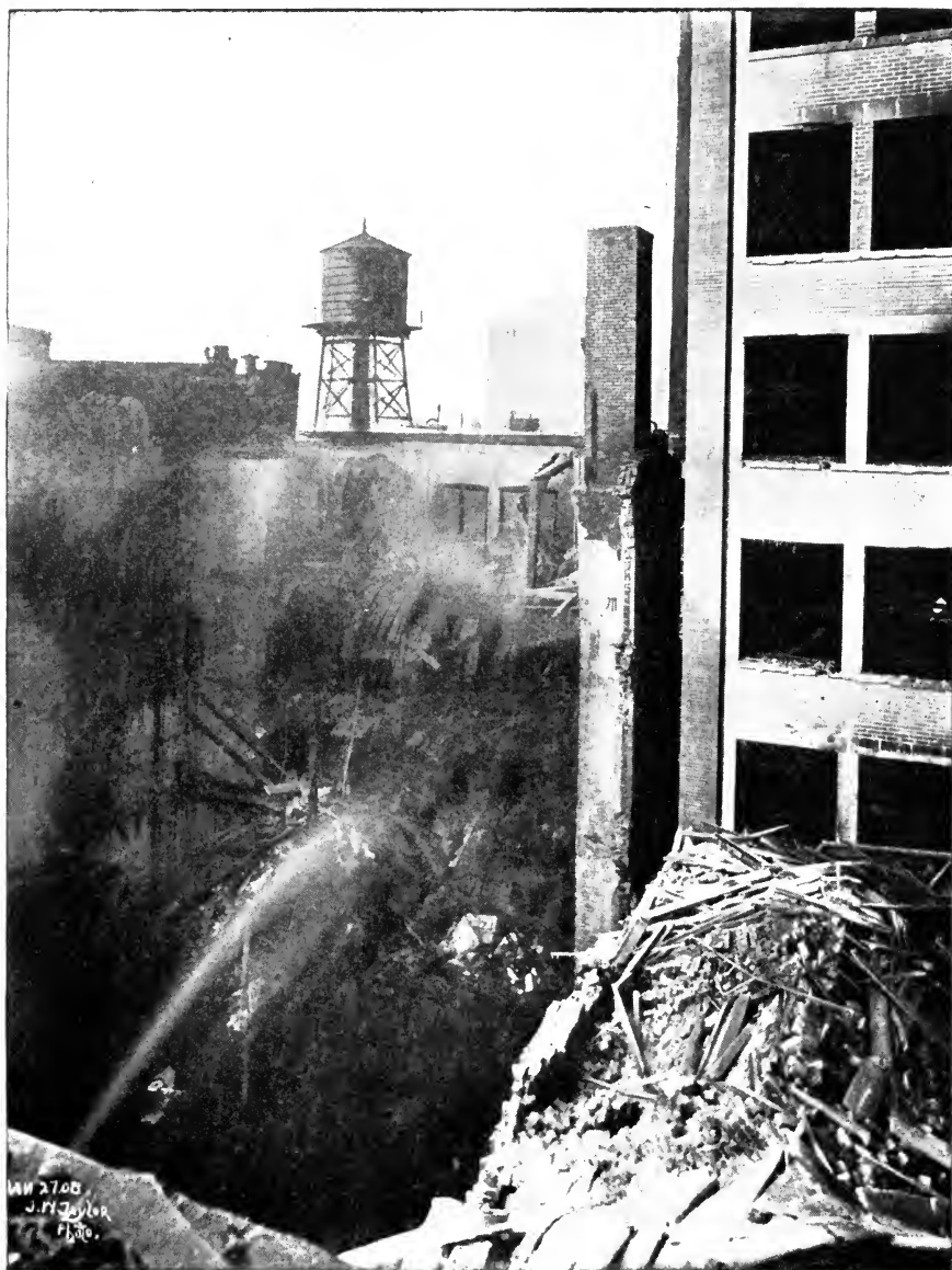
Fig. 49. Alleged "Slow-Burning" Construction This fire lasted 45 minutes.
