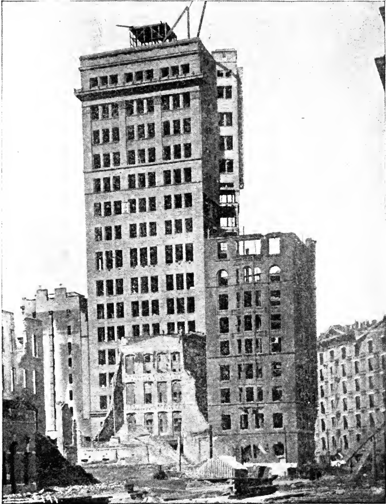
Fig. 10. The Almost Completed Chronicle Building in the San Francisco Fire Nothing in it to burn but a little scaffolding so that it was virtually uninjured
