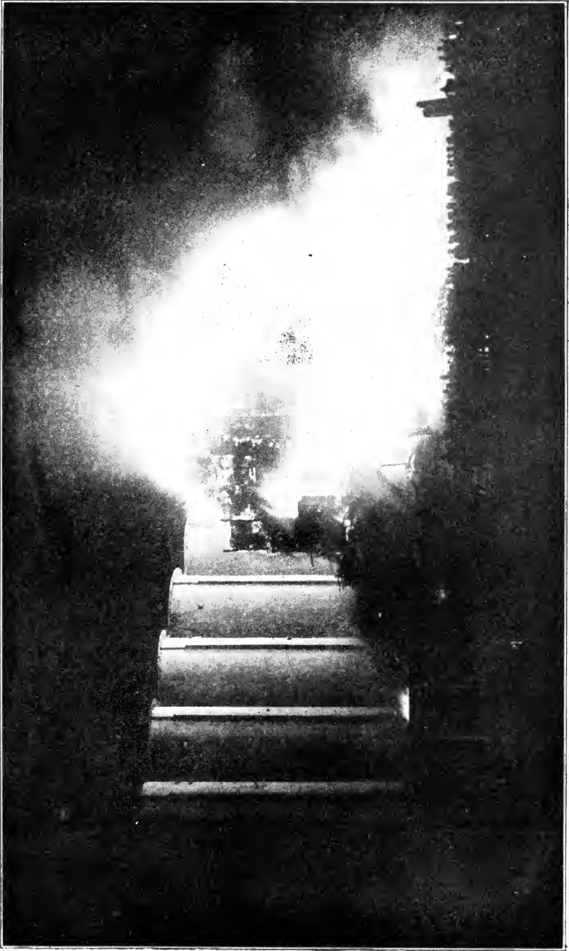
Fig. 99. Destruction of Wooden Elevators of the Peavey Elevator Company. The Concrete Storage Tanks were Uninjured
