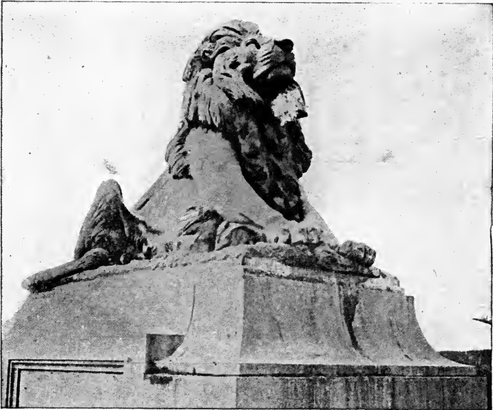
Fig. 42. A Colossal Concrete Lion for a Bridge Approach
