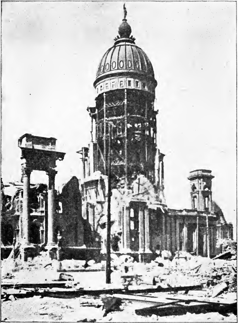
Fig. 31. The Great and Handsome City Hall After the Earthquake and Fire A tile floor had recently been put into the top story and apparently that cut off the fire from destroying the top of the dome.
