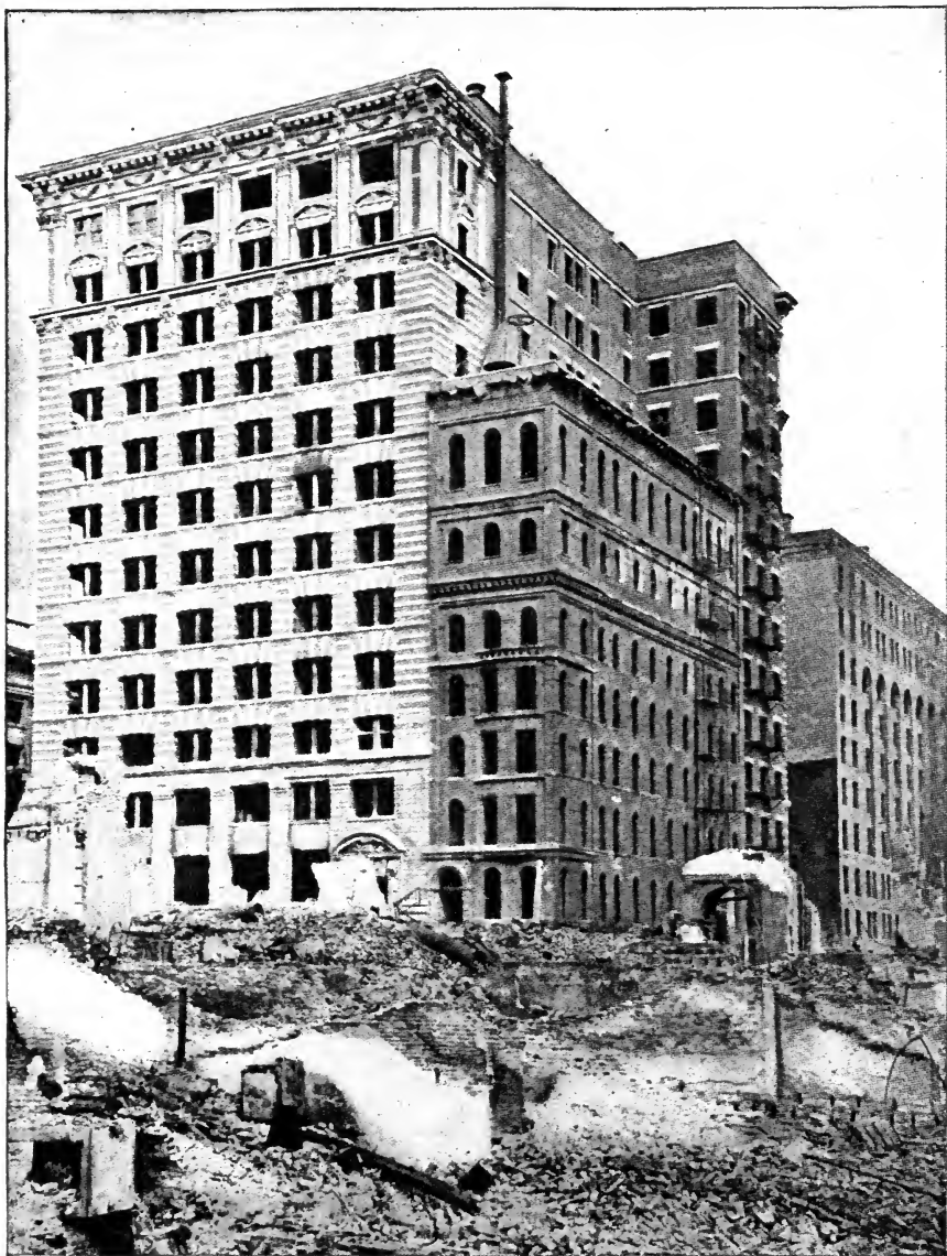
Fig. 13. One of the Big Brick and Terra Cotta Baltimore Buildings after the Fire. The contents gutted but the exterior nearly intact.
