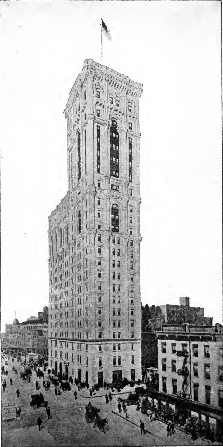
Fig. 20. "The New York Times" Tower. A fine type of office building
