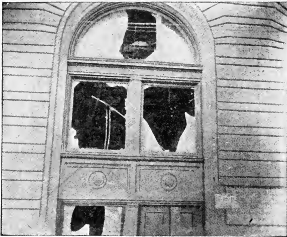
Fig. 23. The Inadequacy of Ordinary Glass Fire went through these windows as it would through paper.
