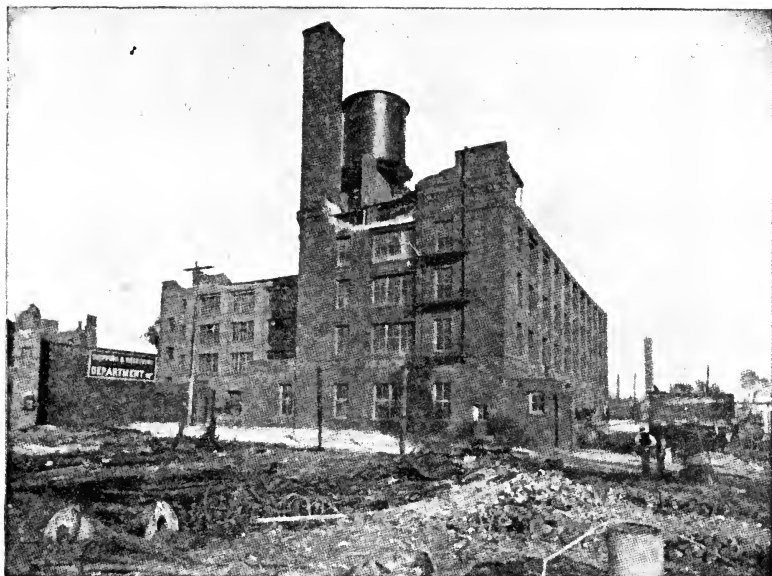
Fig. 34. California Electric Building
