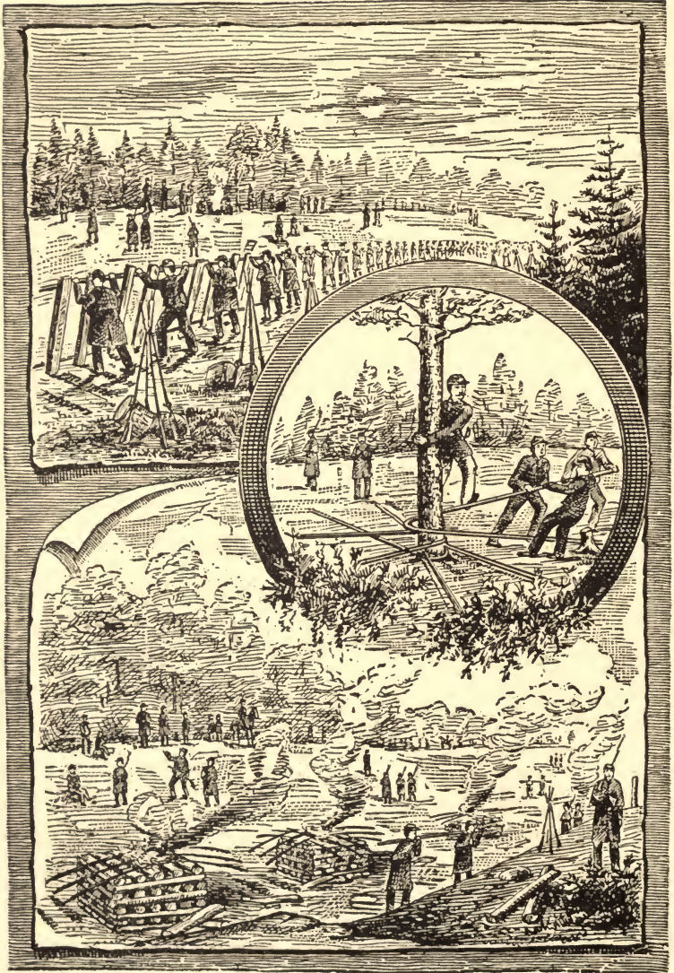
TEARING UP WELDON RAILROAD.
