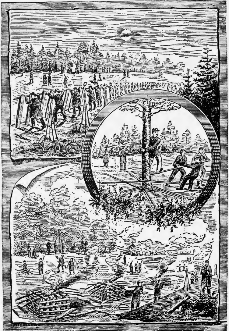
TEARING UP WELDON RAILROAD.
