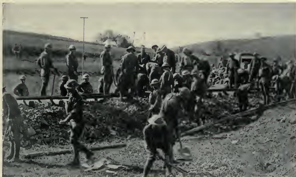
Building Roads in the Recaptured Territory
