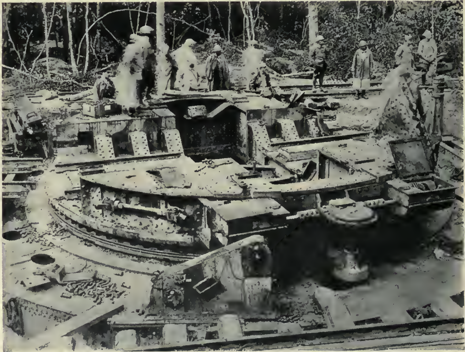
Foundation of One of the "Big Berthas" Which Shelled Paris
