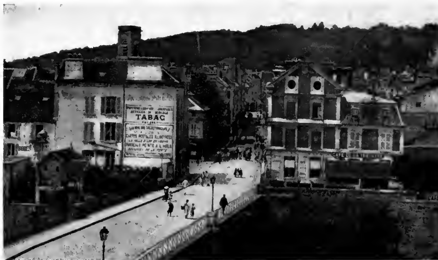
Bridge over the Marne at La Ferte
