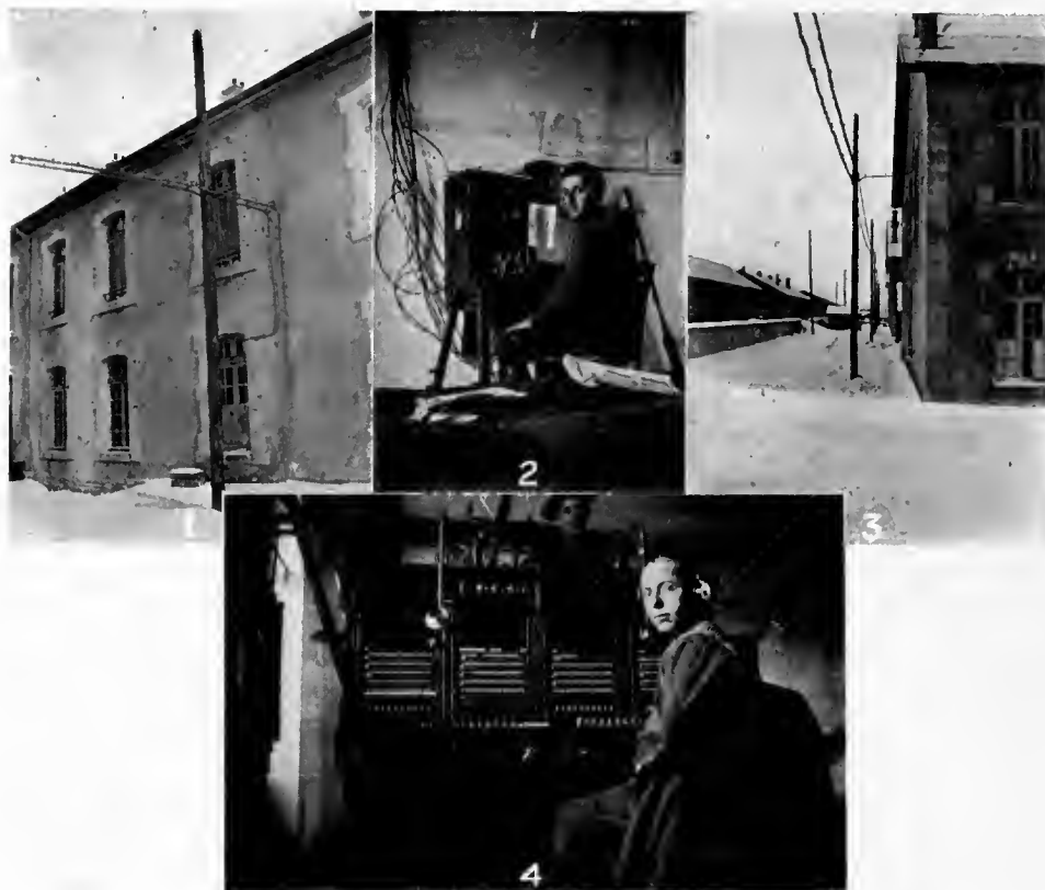
1—Quarters, 2—First Switchboard, 3—Outside Construction, 4—Later Installation.
