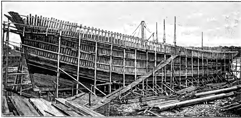
This ship is being built of wood ; many ships are made of plates of iron
