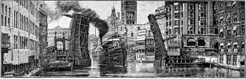
Lifting a bridge in Milwaukee, for a lake steamer to pass
