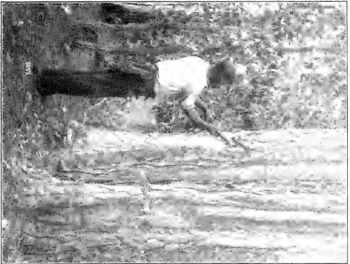
FIG. 65. In a Turpentine Orchard a , chipping, to make a fresh wound; b , "dipping" the "crude," or resin
