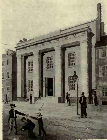
FRANKLIN INSTITUTE, 1825-1922 Seventh Street above Chestnut (East Side)
