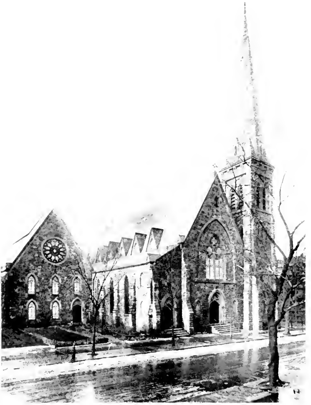
THE PRESENT CHURCH BUILDING
