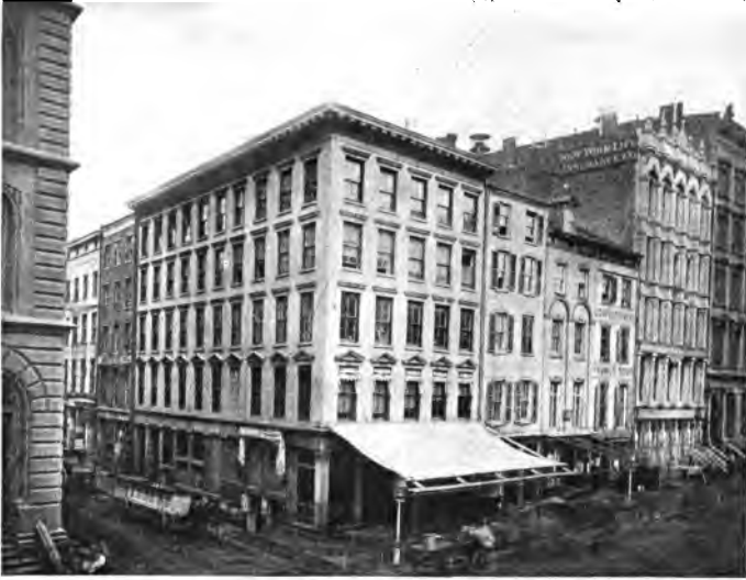
OLD BUILDINGS DEMOLISHED TO MAKE WAY FOR THE EQUITABLE BUILDING
