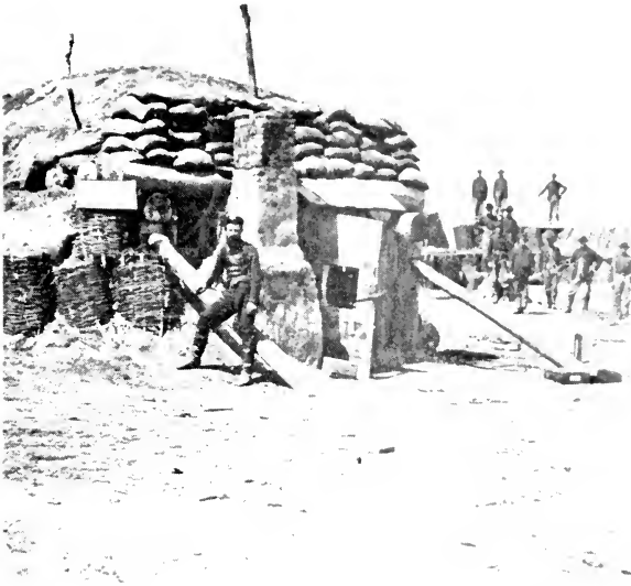
Bomb Proof in Fort Hell. Top of chimney knocked off by a shell. Sticks in top standing in holes made by mortar shells.
