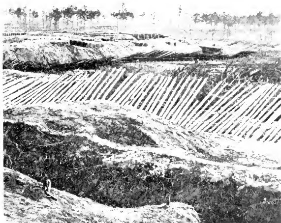
Fort Hell and the ditch with abatis in front of it, taken from where we went out to picket line, showing chevaux-de-frise and ditch, which still remains.
