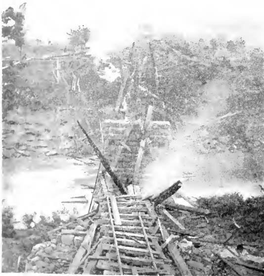
DESTROYING RAILROAD BRIDGE, NORTH ANNA RIVER.
