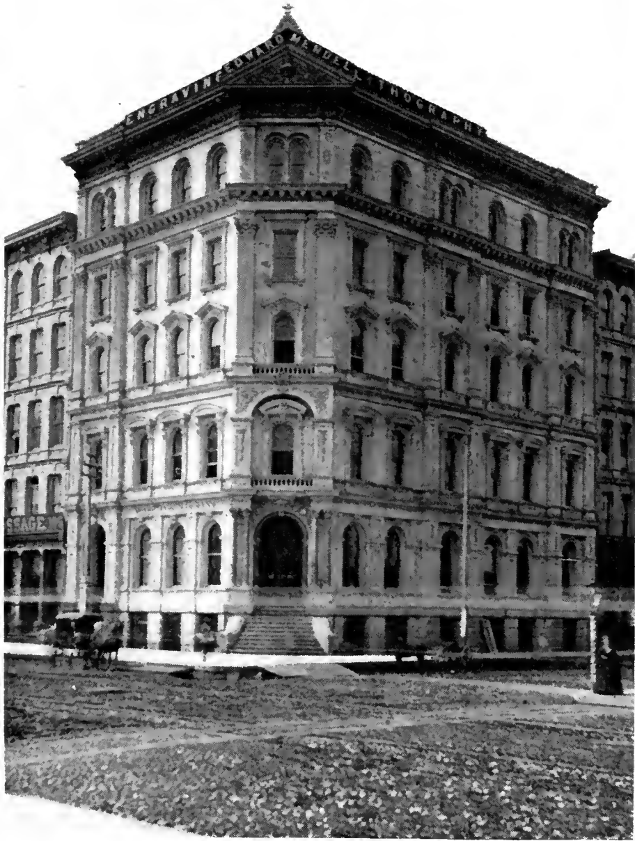
THE BANK'S SECOND BUILDING Southwest Corner State and Washington Streets
