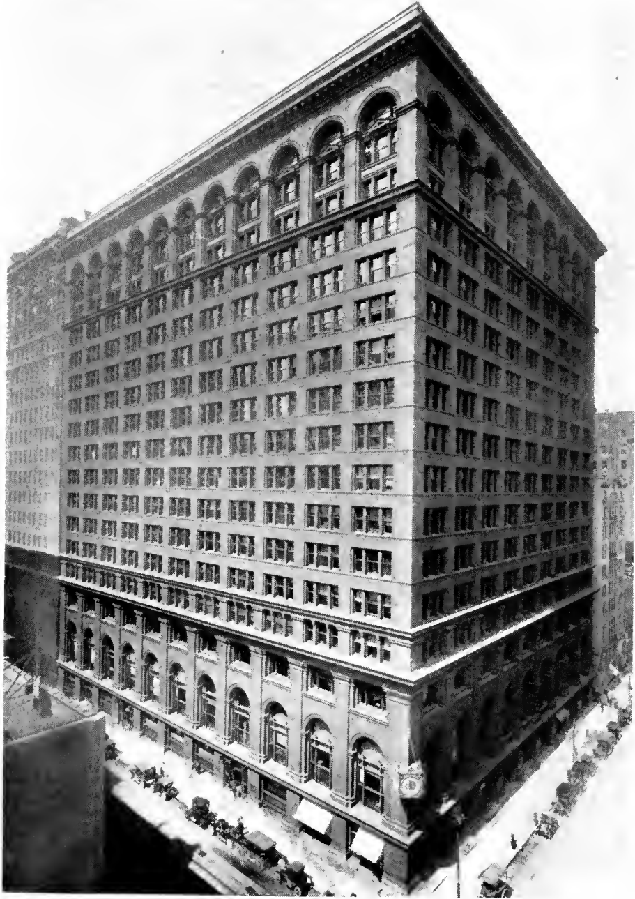
FIRST NATIONAL BANK BUILDING Northwest Corner Dearborn and Monroe Streets
