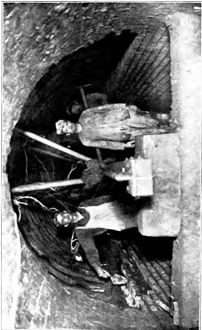
HEADING IN SEWER TUNNEL IN WEST ROXBURY BUILT IN QUICKSAND BY PNEUMATIC PROCESS.
