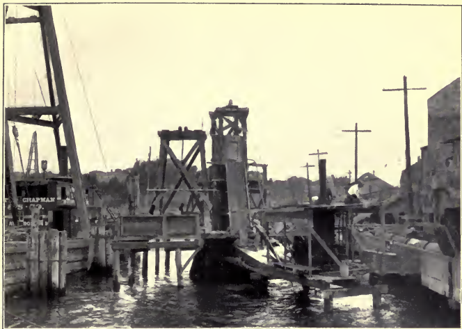
MYSTIC RIVER TUNNEL EXTENSION — SINKING SHAFT AT CHARLESTOWN END OF TUNNEL.
