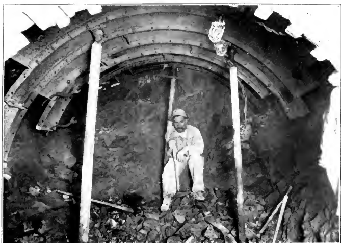
MYSTIC RIVER TUNNEL EXTENSION — HEADING IN ROCK IN TUNNEL UNDER THE RIVER.
