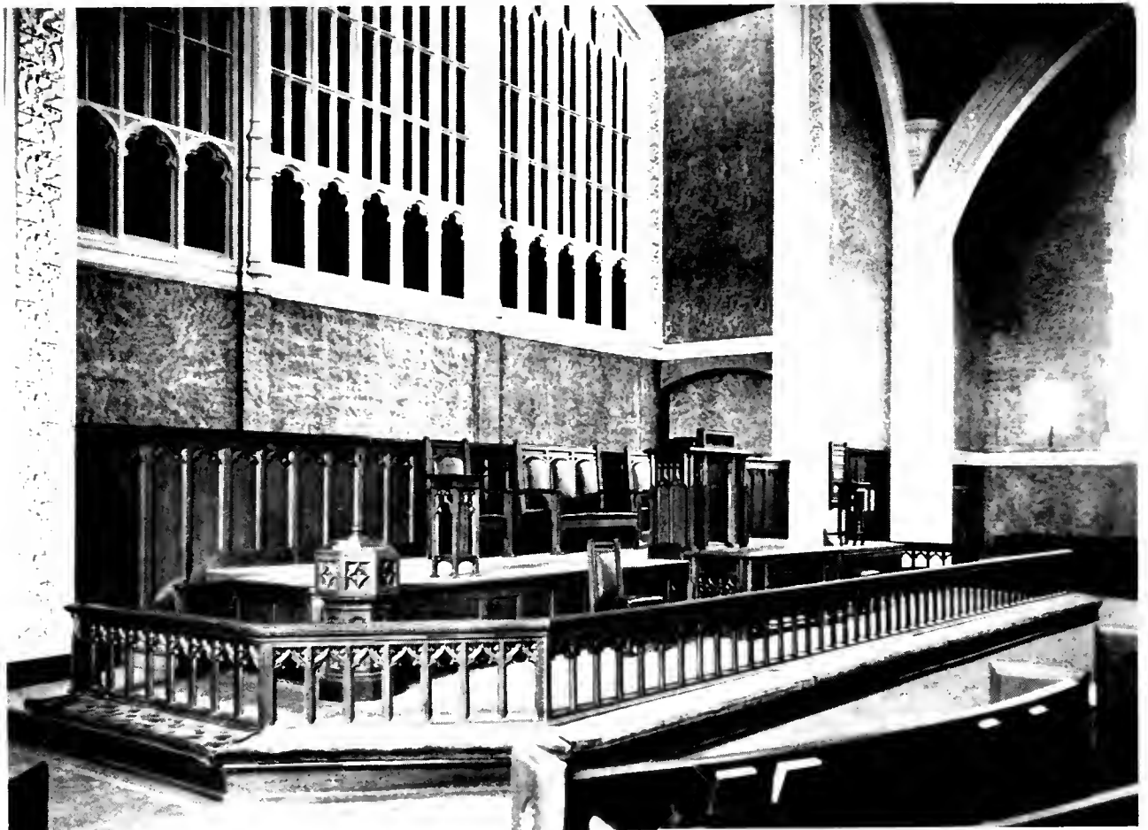
Below, Interior view of sanctuary showing the pulpit area.
