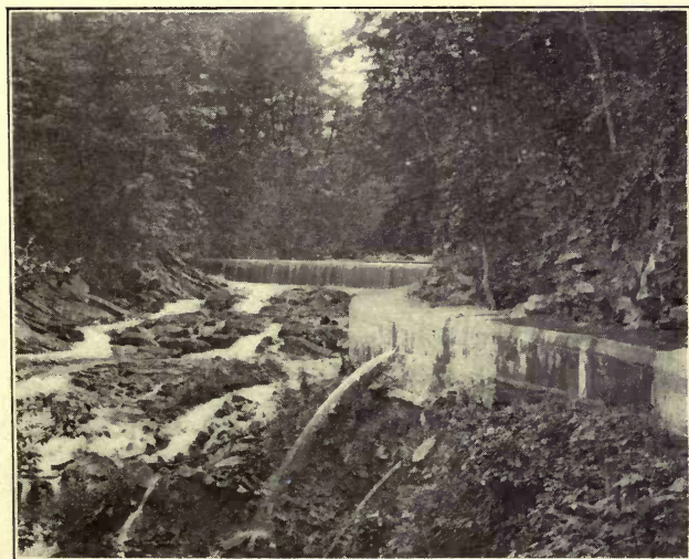
A DAM AND A COVERED RACEWAY.
