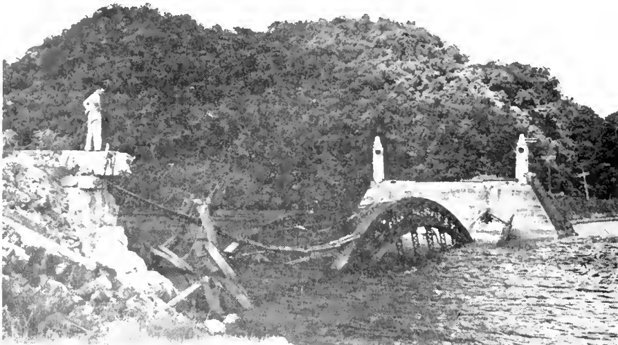
Figure 23... Palau -- Koror. Bombed bridge blocking navigation. July 1946
