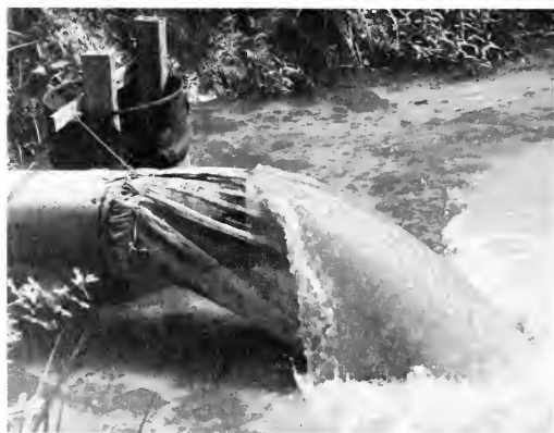
FIGURE 37. Sock-type filters with saran screen for pond inflows. (Diagram from Arkansas Game and Fish Commission; photo courtesy of Fish Farming Experimental Station, Stuttgart, Arkansas.)
