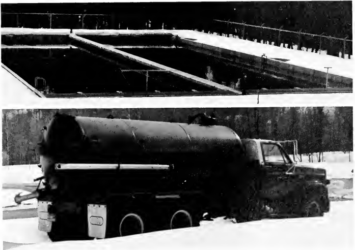
FIGURE 12. Effluent treatment system at the Jordan River National Fish Hatchery consists of two linear clarifiers (top), 30 ft \times 100 ft with a water depth of 4 feet. The system will handle up to 600 gpm divided equally between the two bays. The bays are cleaned by drawing off the top water and moving the sludge with a garden tractor to collection channels. The sludge is then removed with a truck-mounted vacuum liquid manure spreader (bottom). (FWS photos.)
