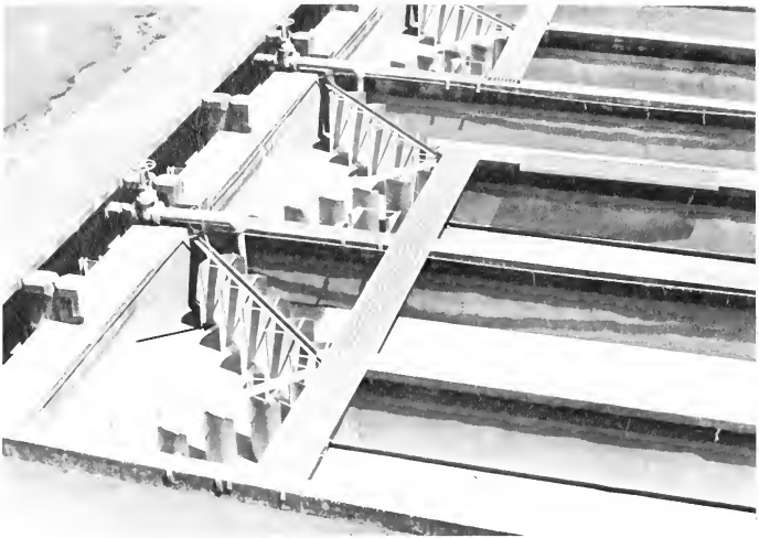
FIGURE 20. Rectangular circulation rearing pond ("Burrows pond"). Water is recirculated around the pond with the aid of turning vanes (arrow). Waste water flows out through floor drains located in the center wall (not shown). (FWS photo.)
