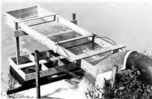
FIGURE 38. Box-type filters mounted in fixed positions. (Diagram from Arkansas Game and Fish Commission; photo courtesy of Fish Farming Experimental Station, Stuttgart, Arkansas.)
