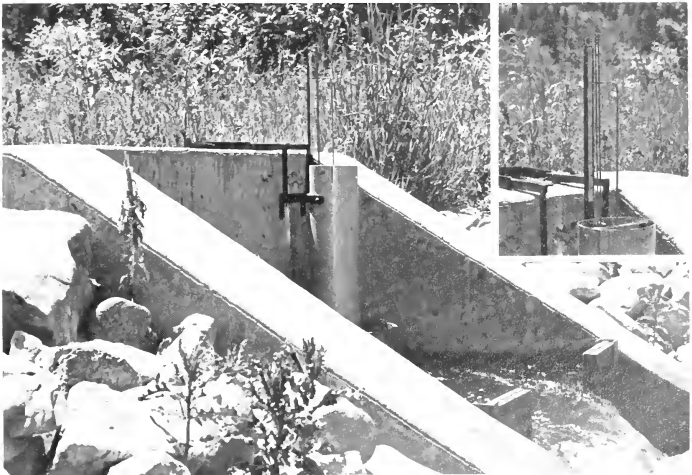
FIGURE D-1. (Top) Diagram of a Cippoletti weir plate. It should be cut from No. 8 or No. 10 galvanized iron plate. The trapezoidal notch must be cut to the exact dimensions as shown. Flow rates with this weir will be twice the values shown in Table D-1. (Bottom) A rectangular weir installed to measure water flow at the discharge of a fish hatchery. A sight gauge (insert) with a float in an aluminum cylinder is used to measure water depth over the crest of the weir. It must be positioned at a distance at least 2.5 times the depth of the water flowing over the weir.
