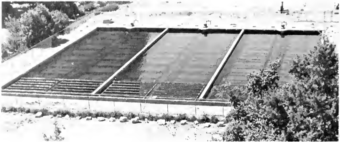
FIGURE 13. Three linear clarifiers located at the Jones Hole National Fish Hatchery, 114 ft \times 41 ft and 6 ft deep. Each unit has a sludge scraper system for sludge removal. These are long redwood boards attached by chain to move and deposit sludge into the sumps at the upper ends of the clarifiers. This system is designed to pump sludge to drying chambers. (FWS photo.)
