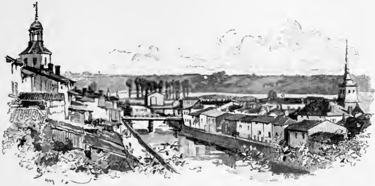
BRIDGE OVER THE AIRE AT VARENNES.
