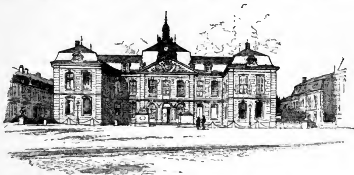
THE TOWN HALL AT SAINTE-MÉNEHOULD.
