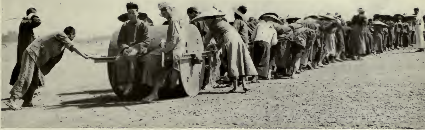
CONSTRUCTION OF AMERICAN AIR BASE IN CHINA. HEAVY ROLLER PULLED BY COOLIE LABORERS PACKS AIRSTRIP. (BELOW) DAILY MENU OF RICE
