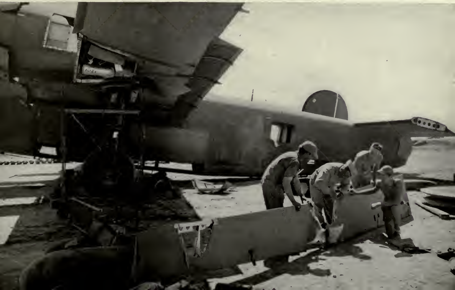
ψ Probing smashed ailerons. After each raid, desert mechanics immediately examine extent of damage suffered by returned bombers.
