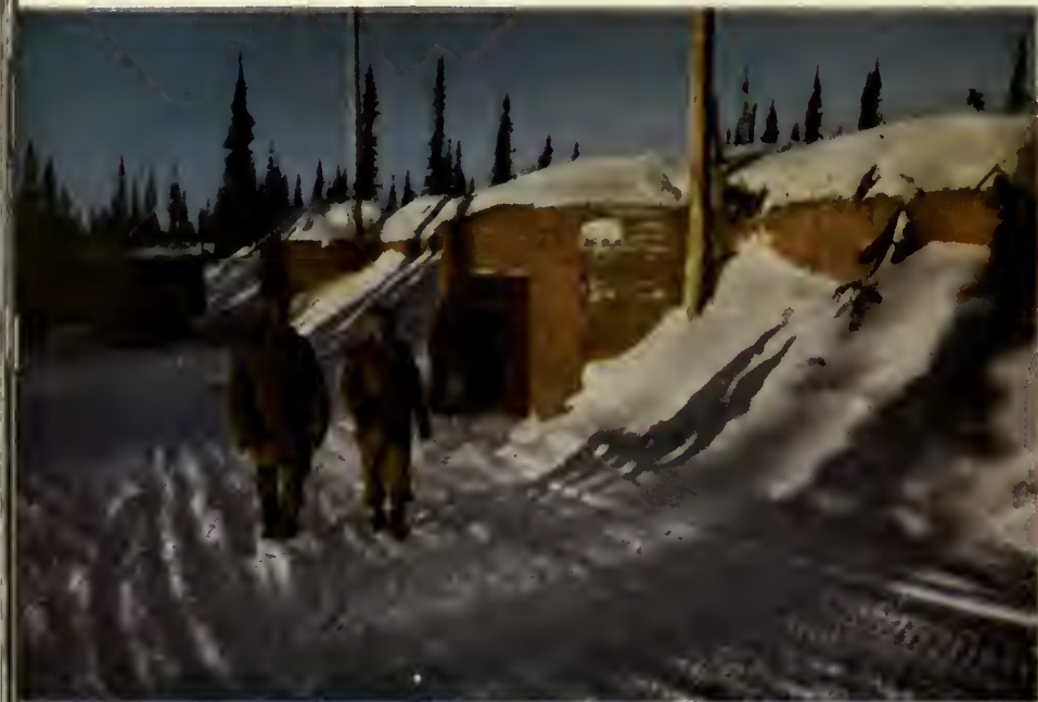
INSULATED ROOT CELLAR PREVENTS FREEZING OF STORED VEGETABLES. (BELOW) TAP ROOM
