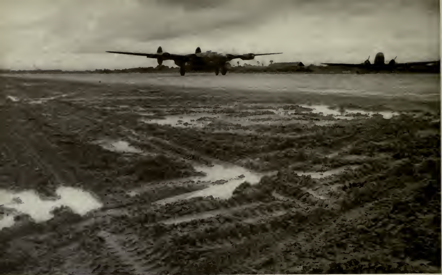
CHABUA. HEAVY SURFACING OVER DEEP MUD OF ONE-TIME RICE PADDIES WAS VITAL IN CONSTRUCTION OF AIR STRIPS. (BELOW) "HEY! PAGE SIR WALTER"
