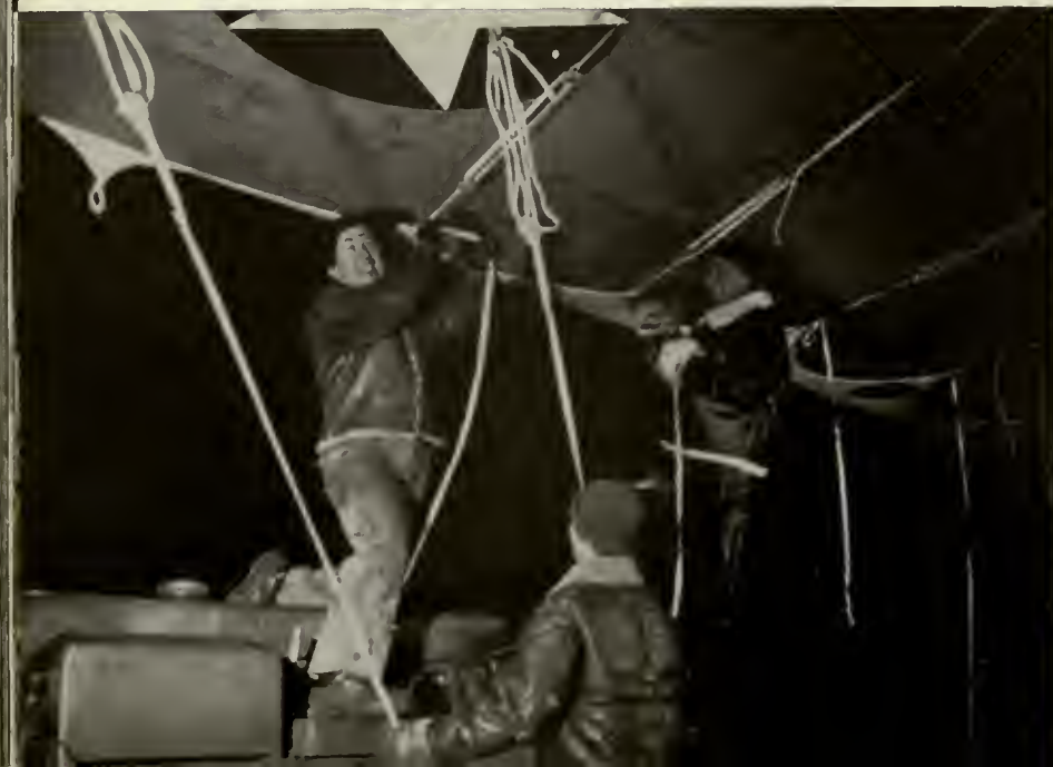
FUSELAGE AND WINGS OF ARRIVING PLANES MUST BE PROTECTED FROM FROST WITH TARPS
