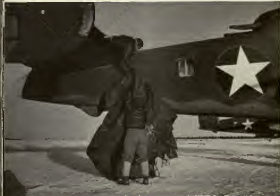
FUSELAGE AND WINGS OF ARRIVING PLANES MUST BE PROTECTED FROM FROST WITH TARPS
