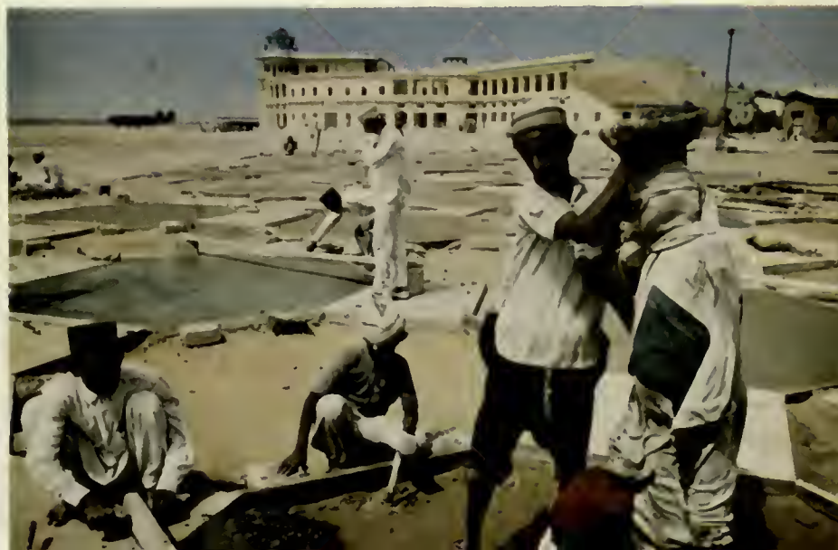
Men place concrete-filled pans upon women's heads and remove them at end of trip. Partially built sections of runway are allowed to dry before last fill.
