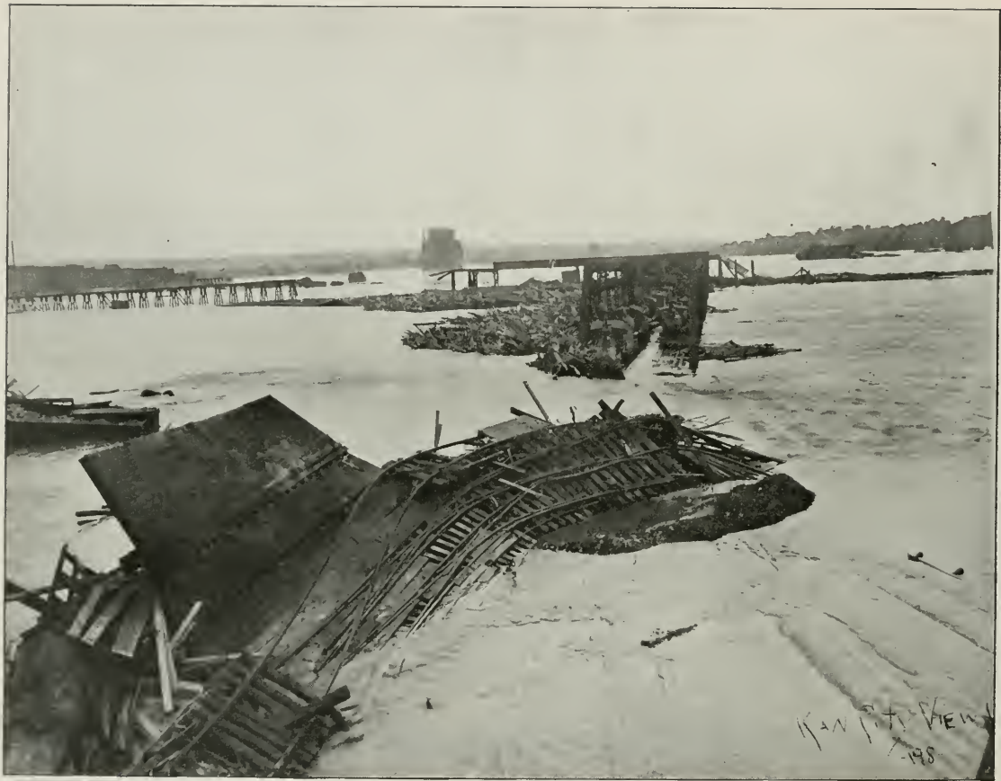
Kansas City, Mo. A break between tracks and bridge.
