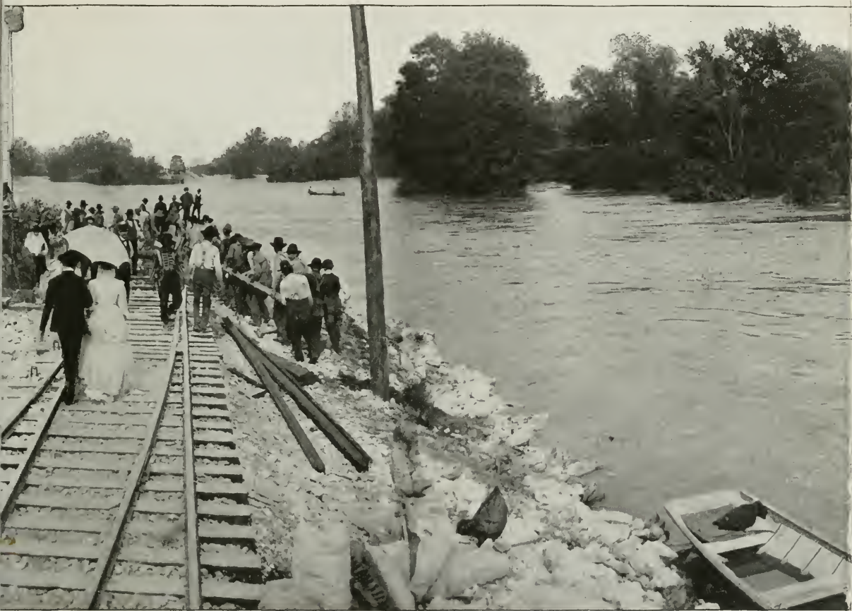
rack of 800 feet, where the water rushed through at a depth of 60 feet.
