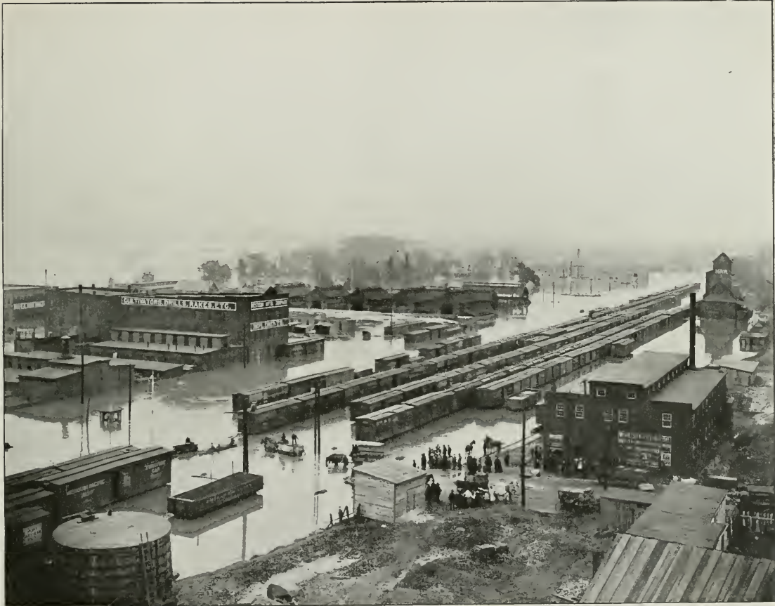
Kansas City, Mo. East Bottoms, at early stage of flood.
