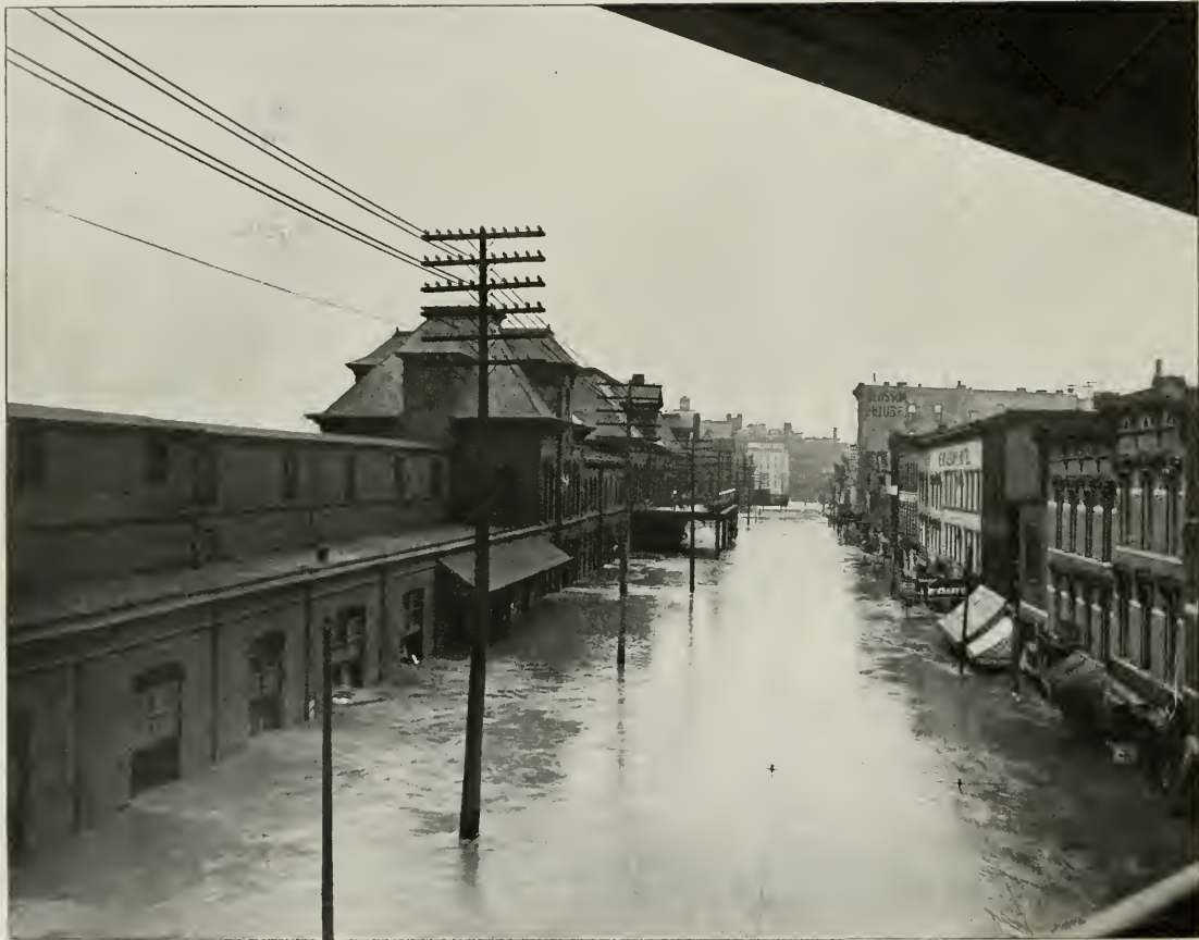
Kansas City, Mo., June 2, 1903. High-water mark in front of Union Passenger Station.
