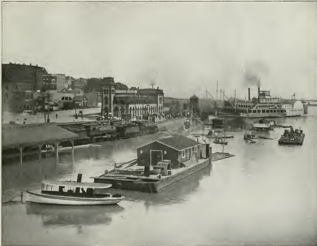
High-water mark at Alton, Ill. C. & A. station and boat landing. Suburban platform, train shed and levee tracks under water in foreground.
