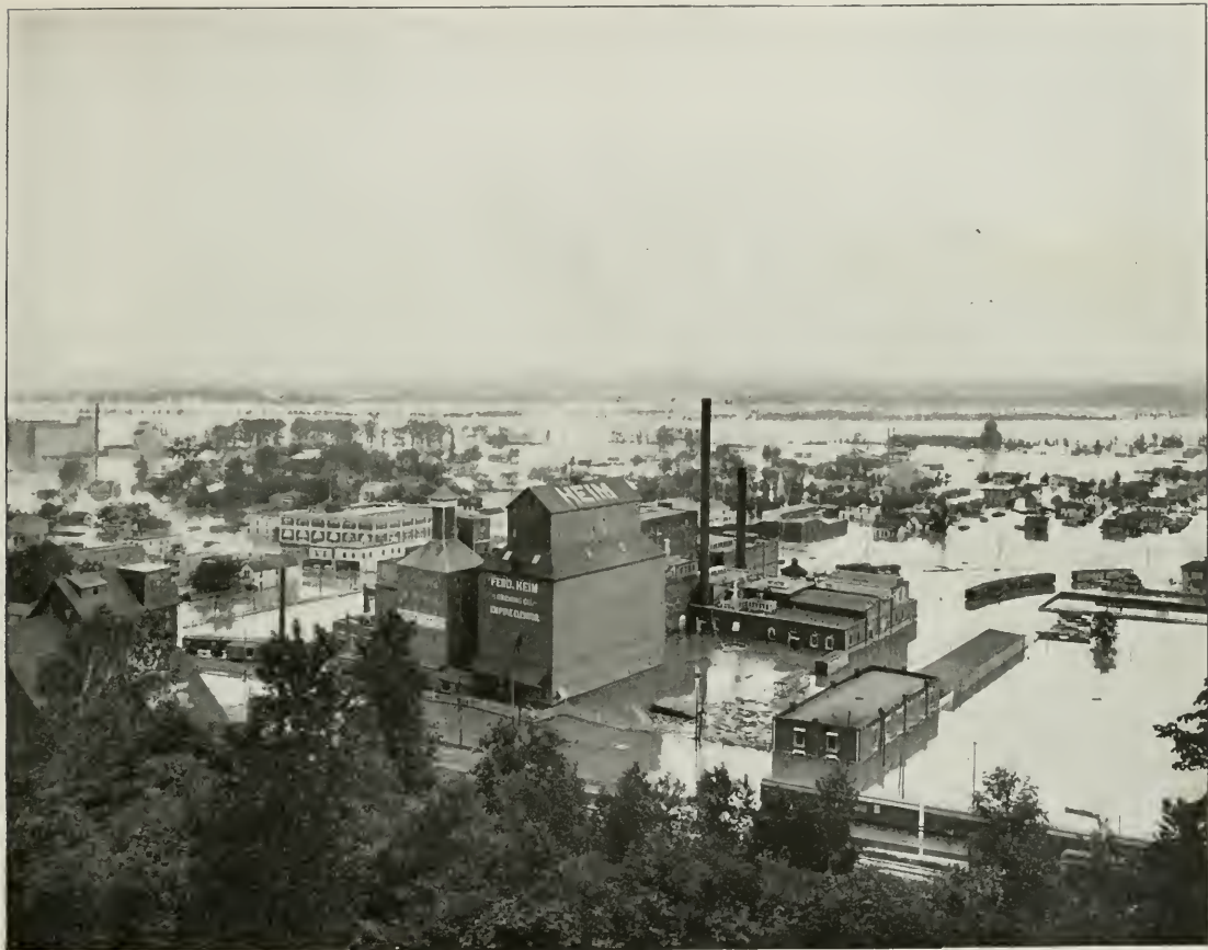
Kansas City, Mo. Submerged district along C. & A, right of way.
