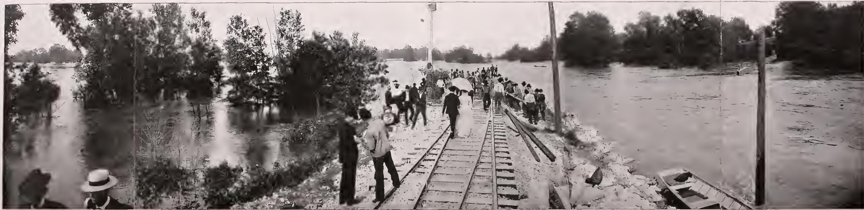
Break in the "Sny Levee," east of Louisiana, Mo., showing break in track of 800 feet, where the water rushed through at a depth of 60 feet.
