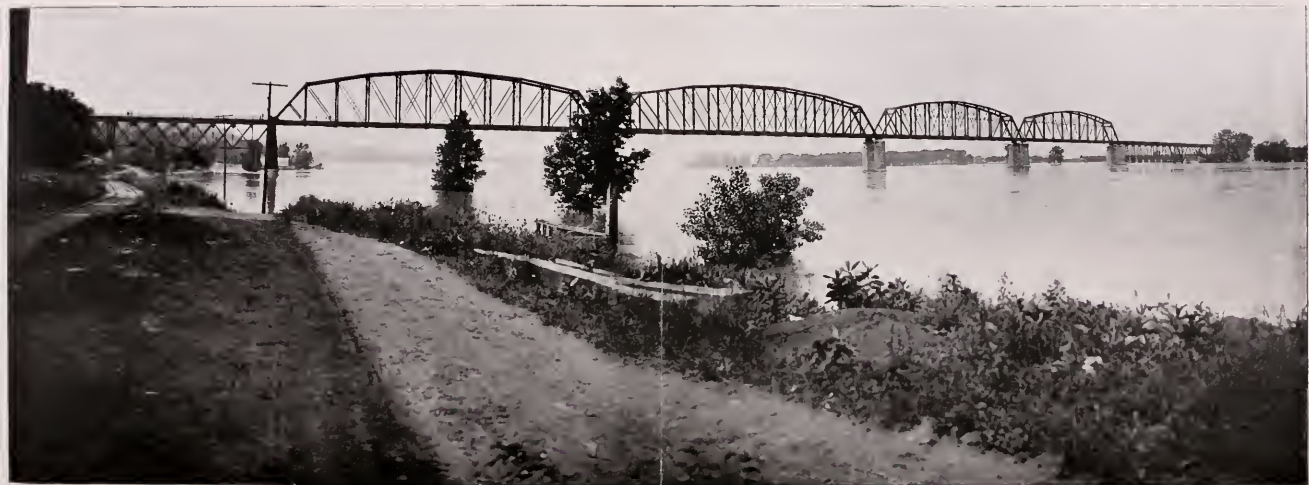
C. & A. New Steel Bridge, Glasgow, Mo., (cost $1,000,000), which stood like a rock against the raging torrents.
