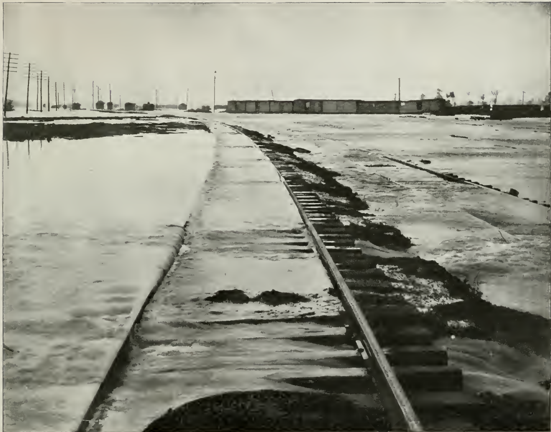
Railway yards at Granite City. Water gradually creeping up over the tracks.
