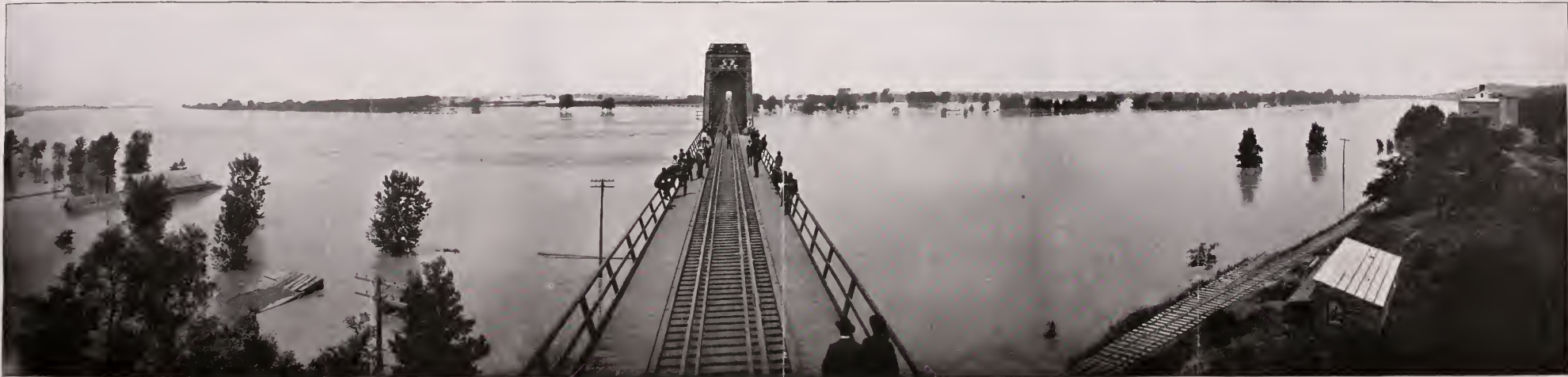
Glasgow, Mo., and the Great Steel Bridge over the Missouri, showing submerged farm property on river front.
