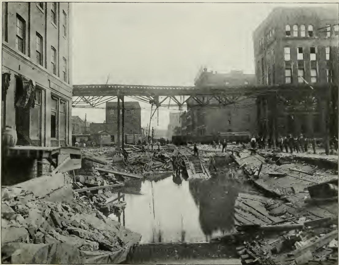
Kansas City, Mo. Sink hole on Santa Fe Street, two blocks from the Missouri River.
