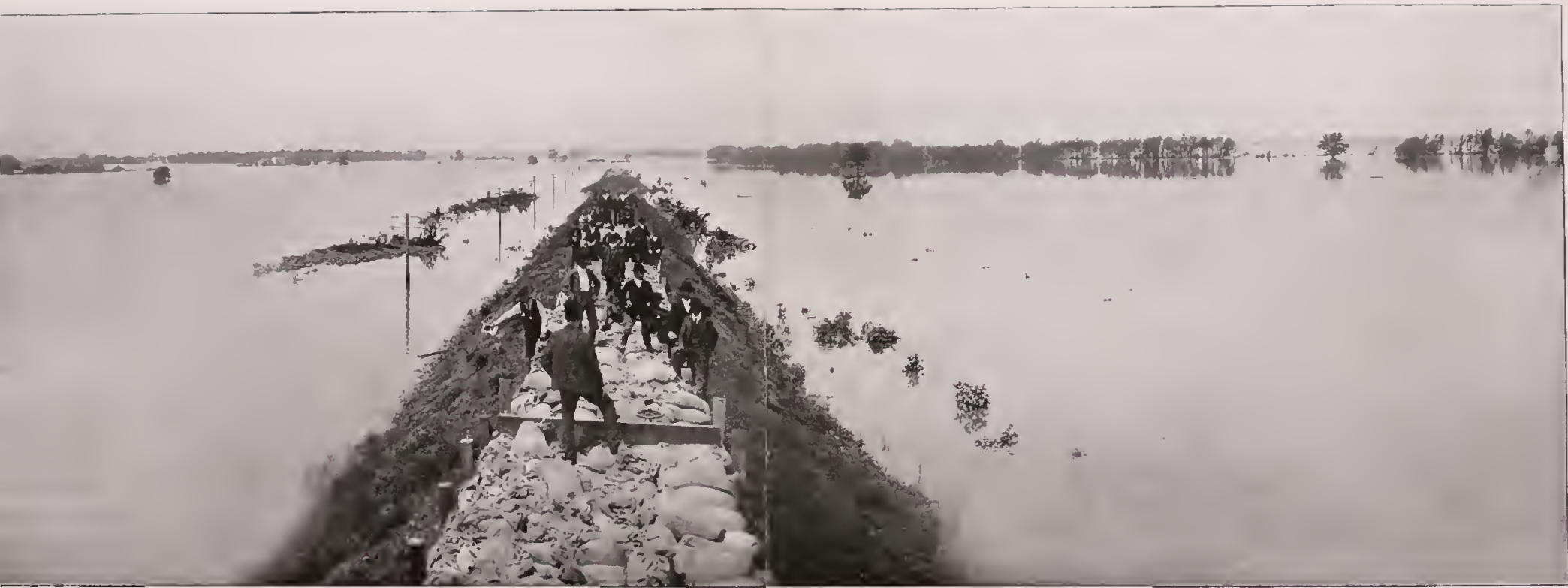
Glasgow, Mo., west of C. & A. Bridge. A work train distributing "sand bags" in an effort to save the railway embankment and track. Beyond the point where the tracks go under the water a lake twenty miles in circumference was formed by the back waters of the Missouri River.
