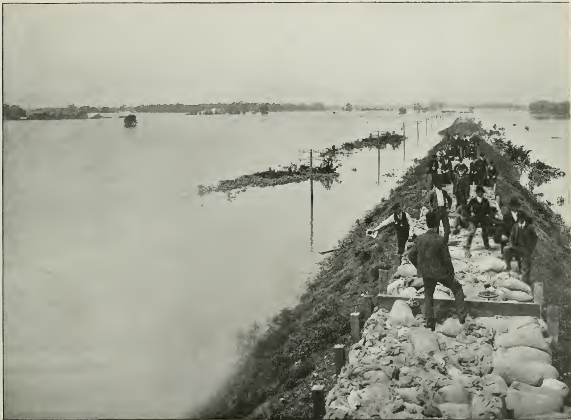
Glasgow, Mo., west of C. & A. Bridge. A work train distributing "sand bags" in an effort to save miles in circumference was formed by
