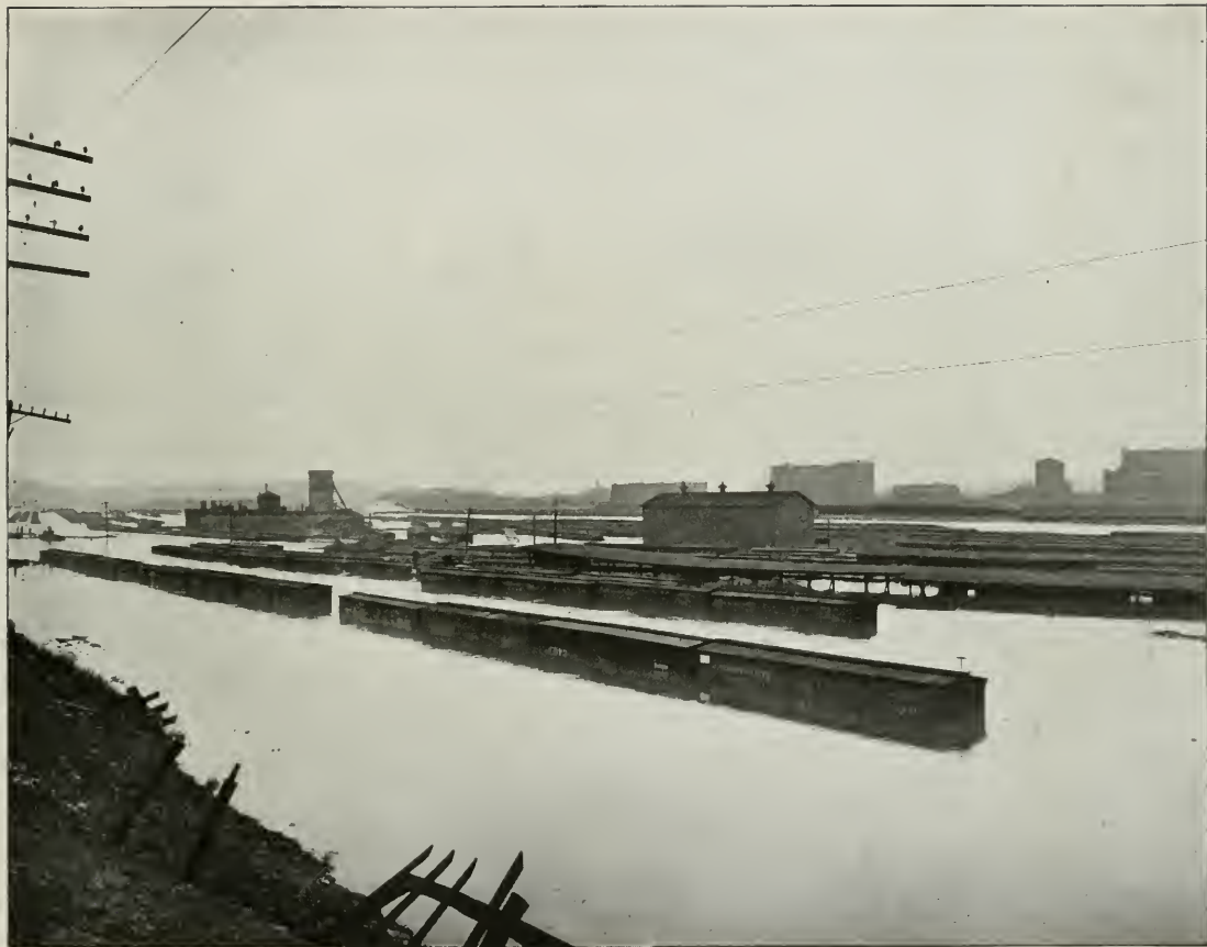
Kansas City, Mo., June 1, 1903 High-water mark in Railway Yards C. & A. ice house in foreground.
