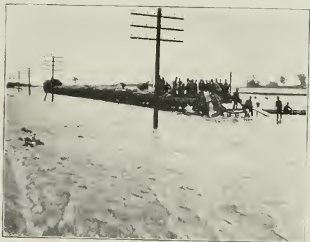
Raising and repairing the track at the end of the break at Granite City.
