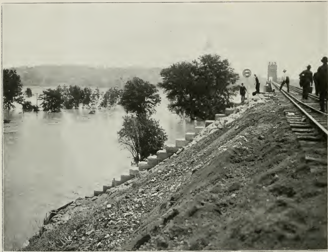
Patrolling and watching the largest bridge abutment in the world, at Glasgow, Mo., to protect it from the rush of the waters.
