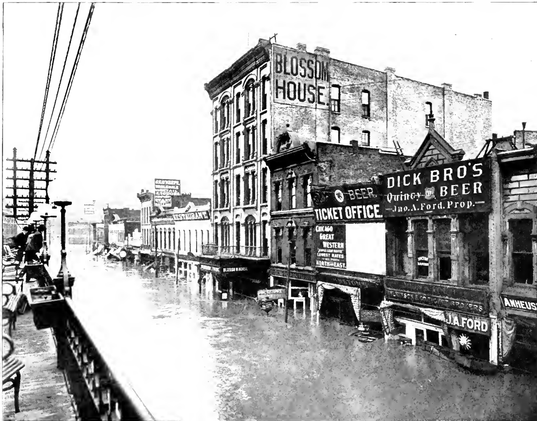
Union Avenue looking west from veranda of Union D-pot, Kansas City, Mo., June 2, 1903. High-water mark
