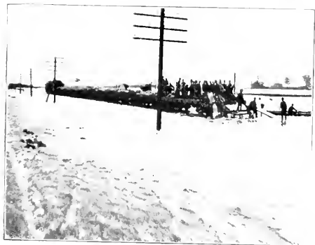
Raising and repairing the track at the end of the break at Granite City.
