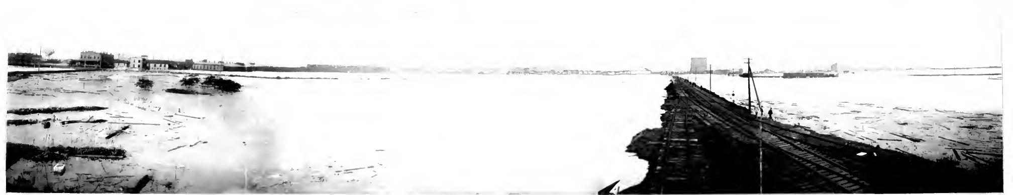
Bird's-eye panoramic view of flooded railway property at East St. L.
