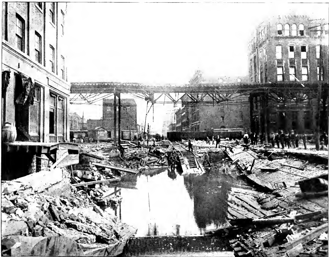
Kansas City, Mo. Sink hole on Santa Fe Street, two blocks from the Missouri River.
