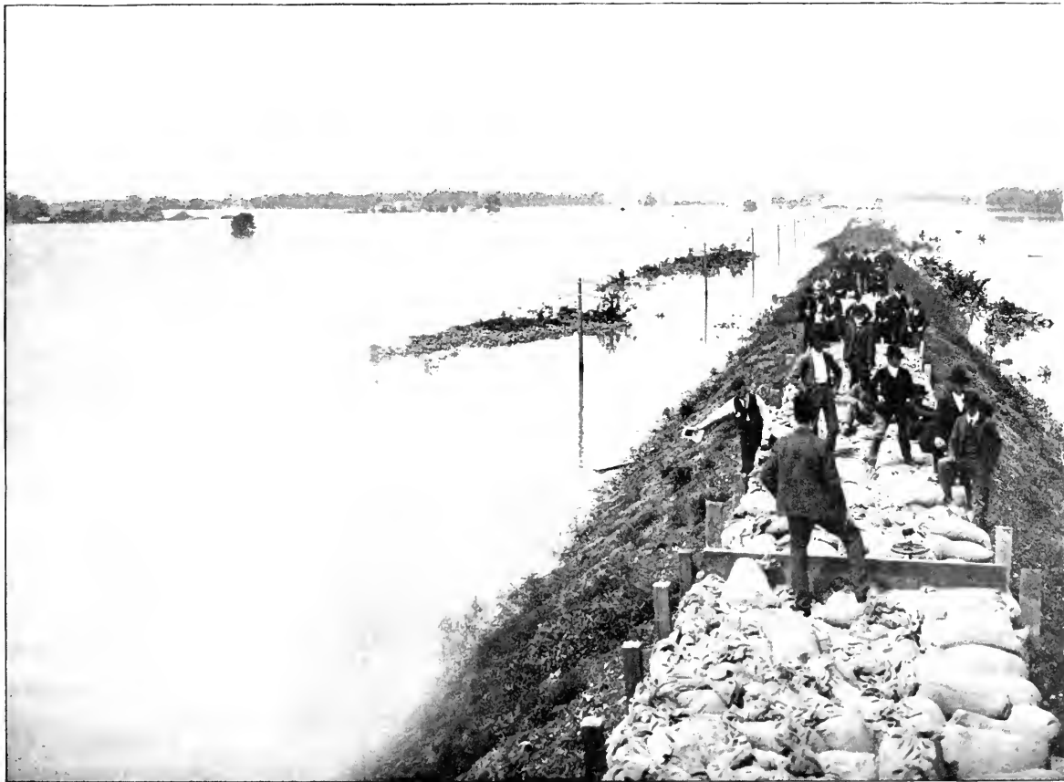
Glasgow, Mo., west of C. & A. Bridge. A work train distributing "sand bags" in an effort to save th miles in circumference was formed by
