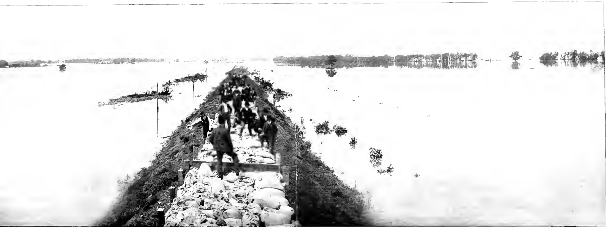
Glasgow, Mo., west of C. & A. Bridge. A work train distributing "sand bags" in an effort to save the railway embankment and track. Beyond the point where the tracks go under the water a lake twenty miles in circumference was formed by the back waters of the Missouri River.
