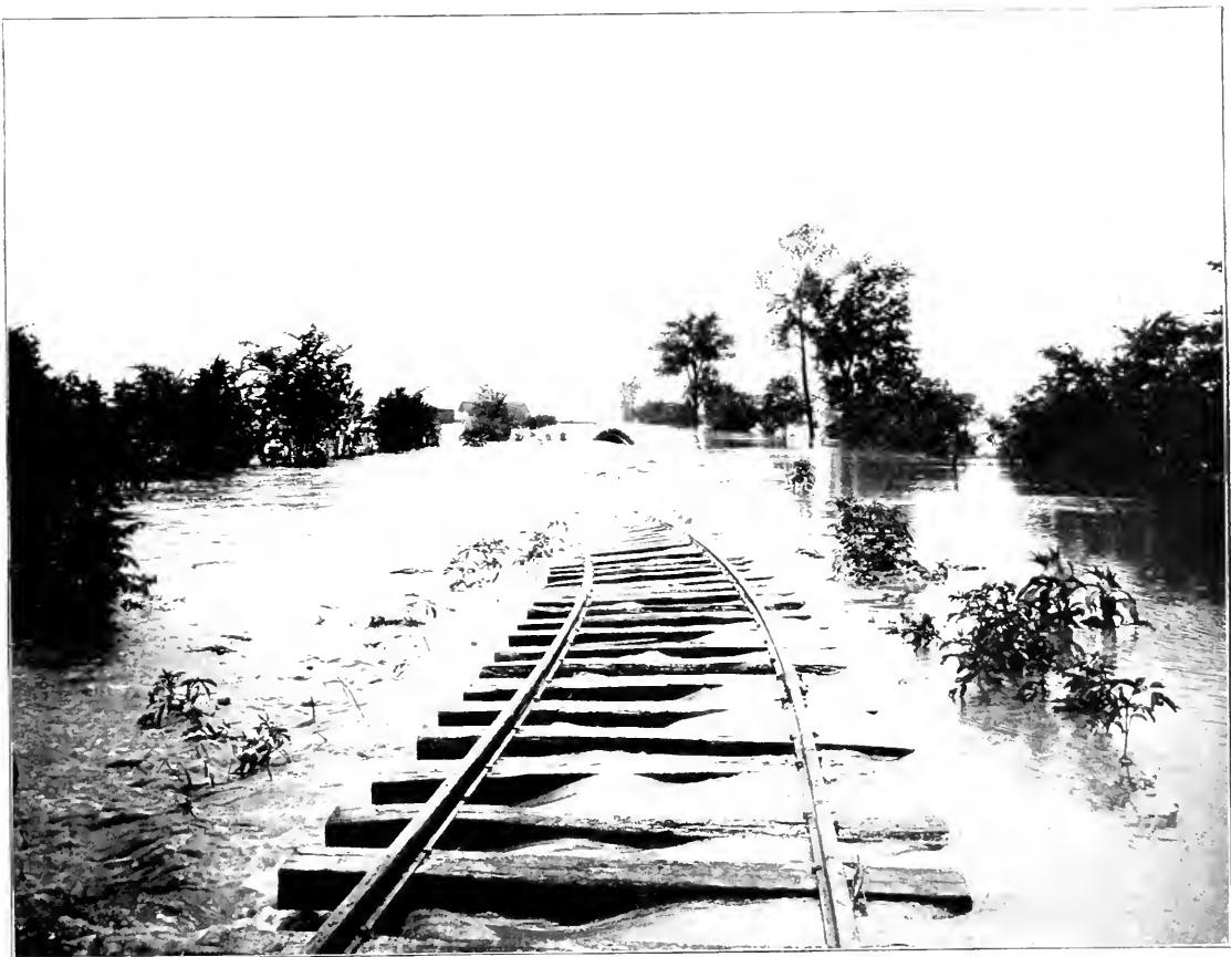
Cedar City, Mo., the terminus of C. & A. track, on the South Branch.
