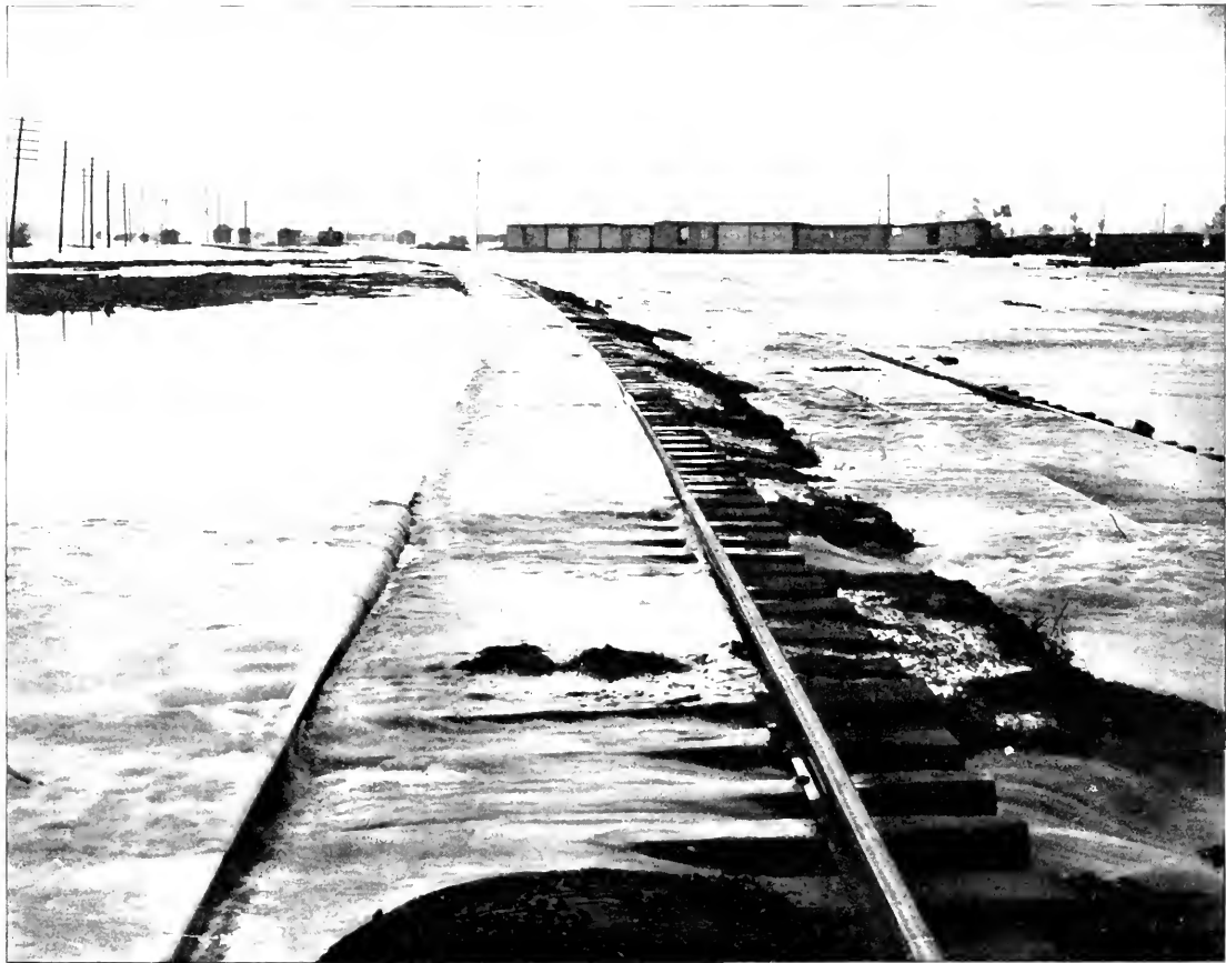
Railway yards at Granite City. Water gradually creeping up over the tracks.
