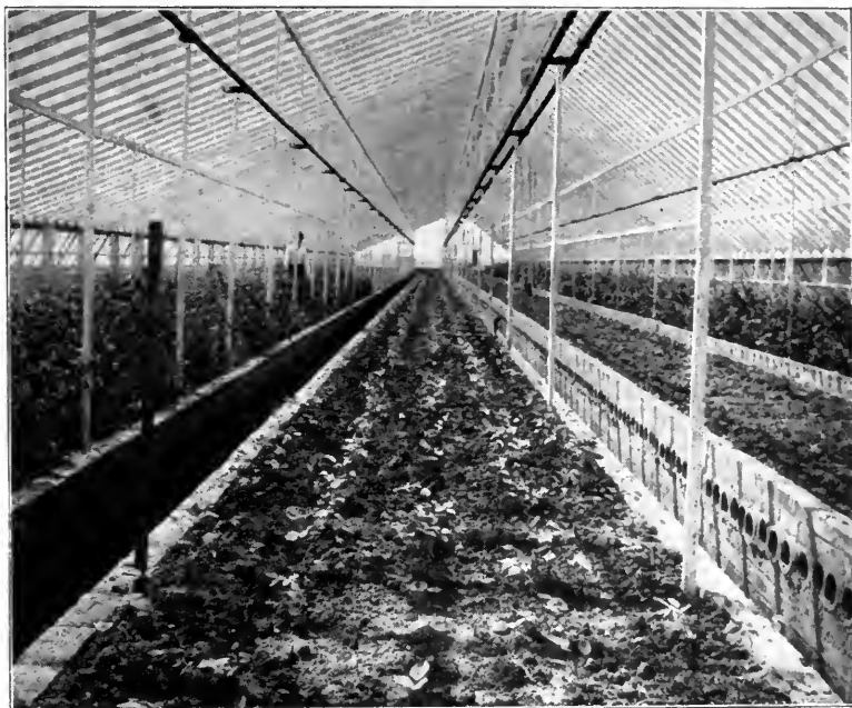
Rose House, Showing Bench Construction, Brick Walls with Tile Bottoms.
