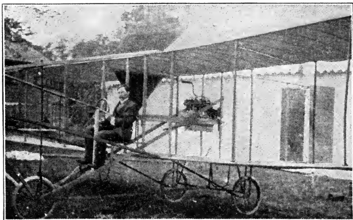
Position of Motor on Brauner-Smith Machine.
