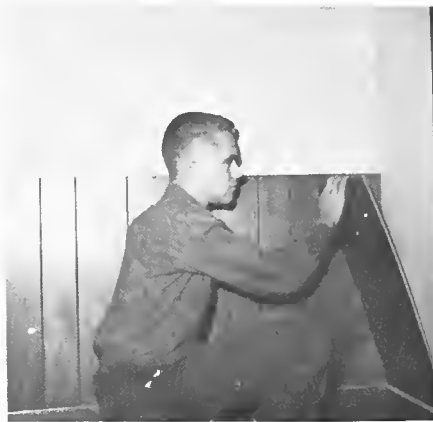
Cutting and applying wainscoting to walls of President's office
