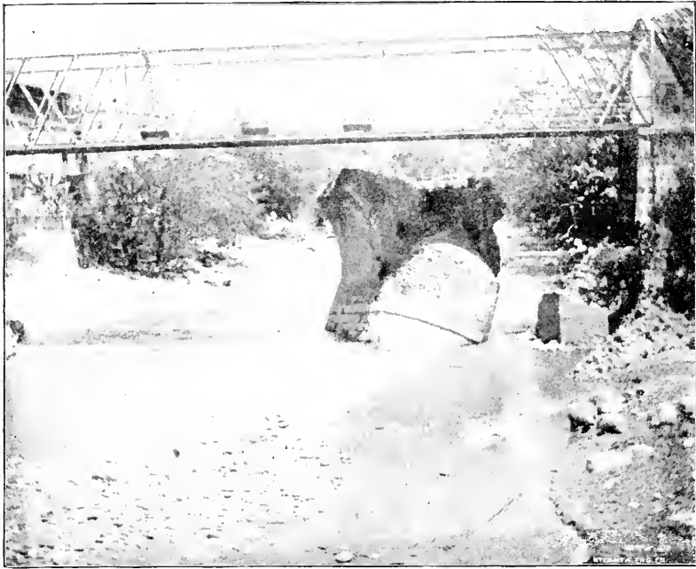
RUINS OF BRIDGE OVER THE GUALÍ DESTROYED BY EARTHQUAKE.
