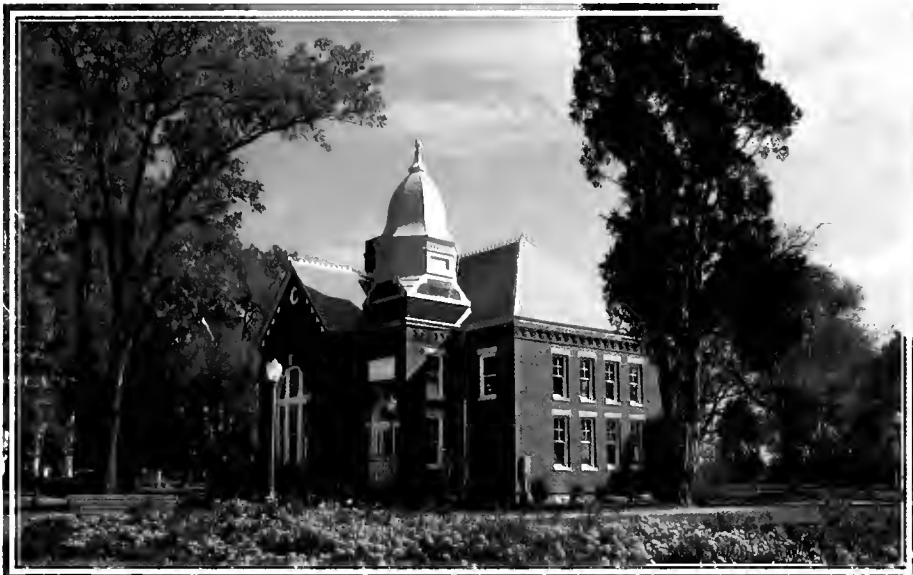
Workers paid close attention to detail when it came to restoring the Center for Campus Ministry. A metal roof and white “dimples” across the top of the building would have been visible features of the building in 1888.
