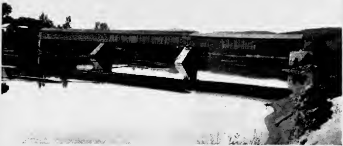
OLD WOODEN CHESHIRE BRIDGE BUILT ABOUT 1800
