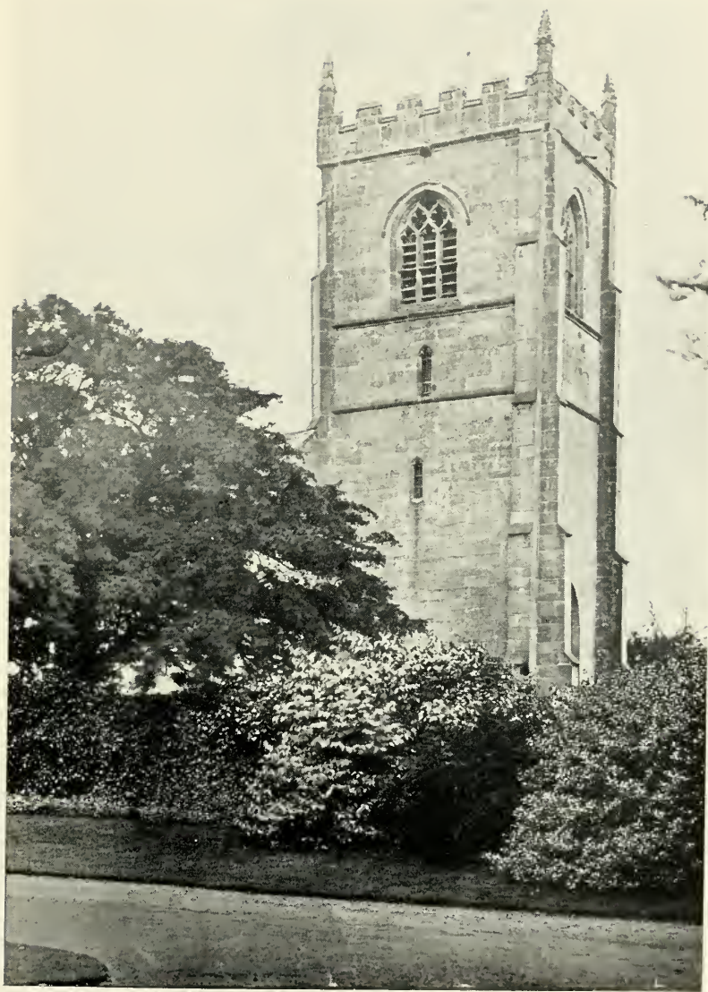
MUCKLESTONE CHURCH TOWER.
