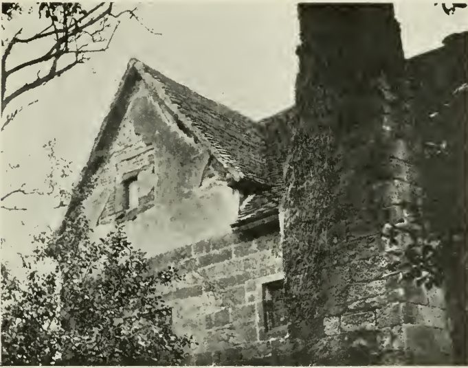
A GABLE AT THE BACK OF MEES HALL.
