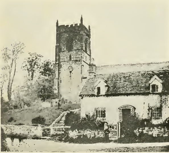
THE CHURCH WITH ADJOINING COTTAGE AS THEY WERE BEFORE THE “RESTORATION.”
