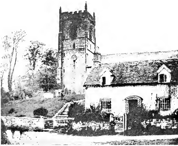
THE CHURCH WITH ADJOINING COTTAGE AS THEY WERE BEFORE THE “RESTORATION.”
