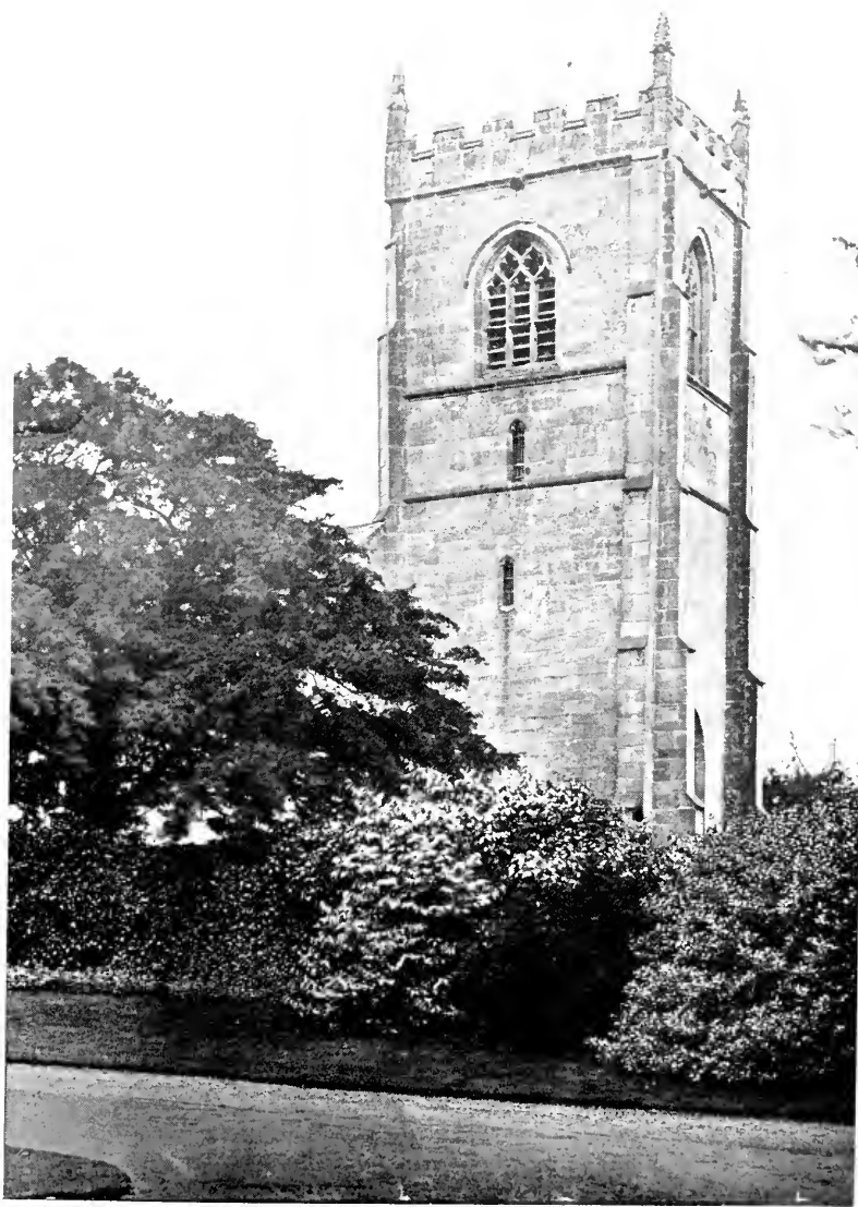
MUCKLESTONE CHURCH TOWER.
