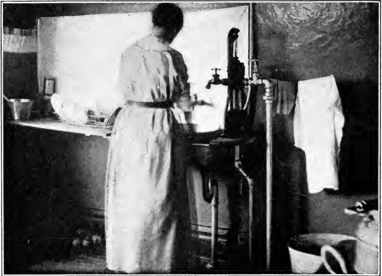
FIG. 60. — Washing dishes. Notice the rack at the left for draining dishes. The sink is too low.
