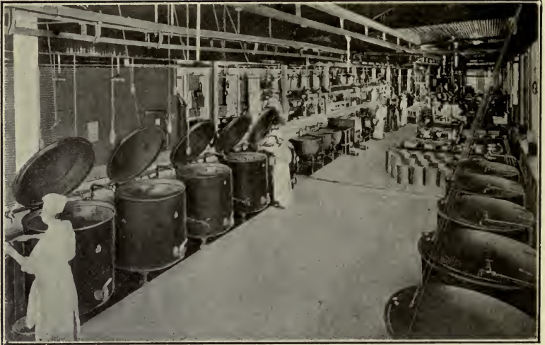
Fig 60.—Stock Boilers. (Courtesy of the Franco-American Food Co.)
