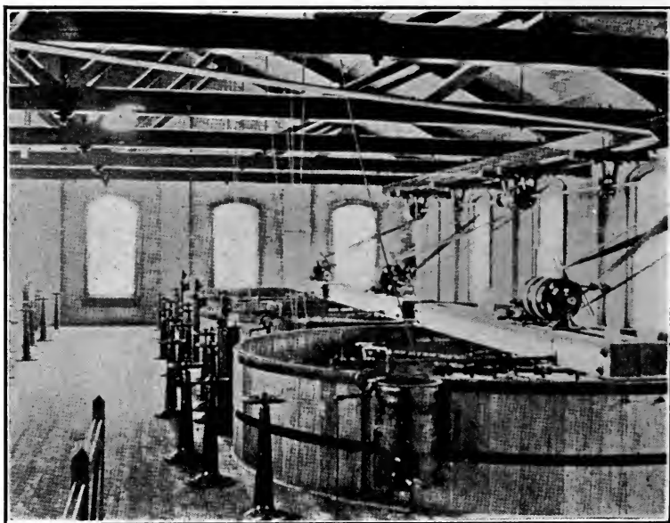
Fig. 2.—View of the Interior of the East Albany, N. Y., Filter-plant. (Courtesy of John Wiley & Sons.)
