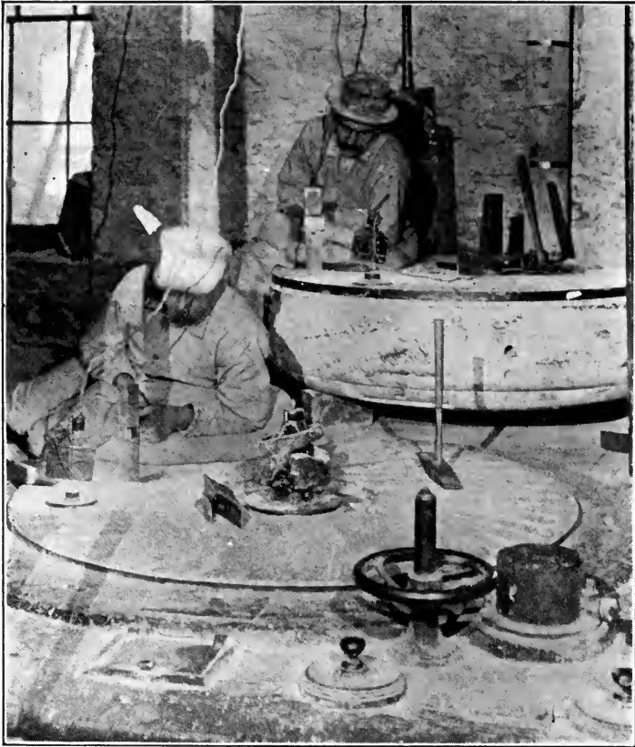
Fig. 9.—Roughening Burr-Stones. (Courtesy of the Washburn-Crosby Co.)
