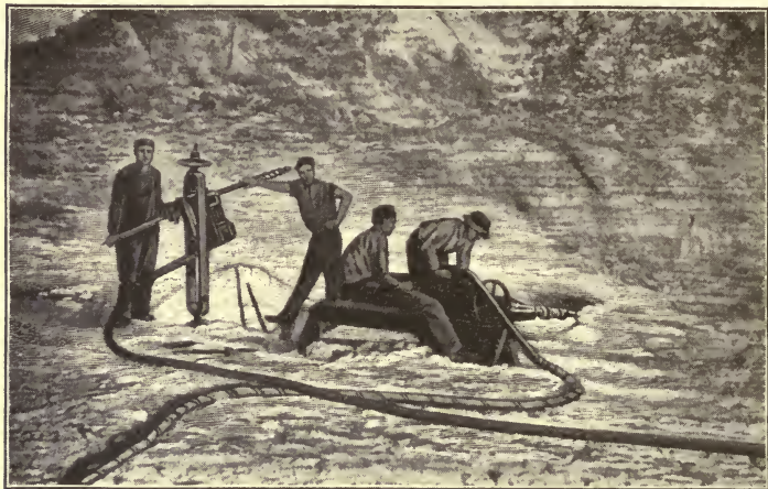
Drilling for blast in a Kansas mine.
