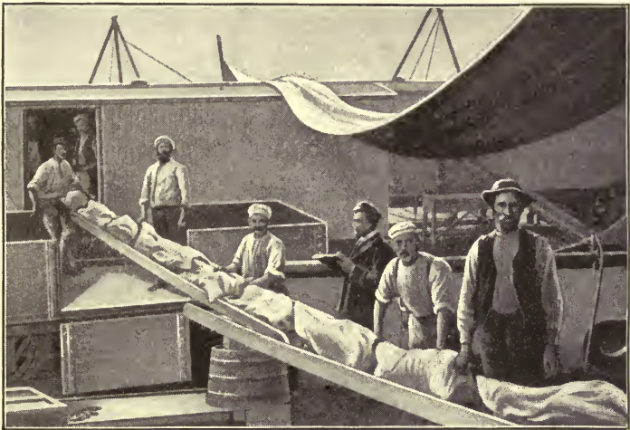
Slide into the cold storage chamber of a steamer.
