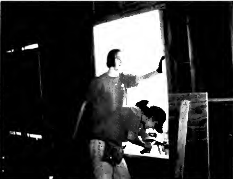
Ann Serdynski and Maggie Vargas work together to build the window frame.
